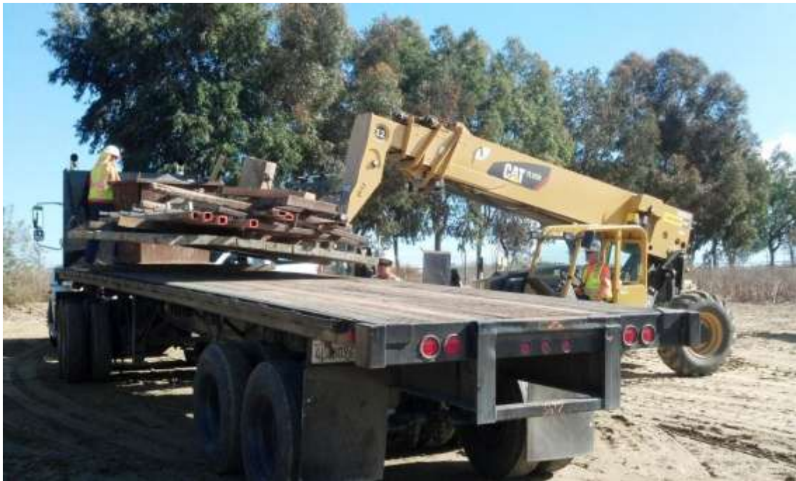
Figure 4: Crews mobilizing equipment at M45-T1, Segment 8, Phase 4.
