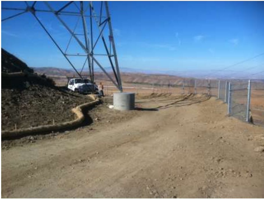
Figure 3: Segment 5 fence installation at Construct 44.
