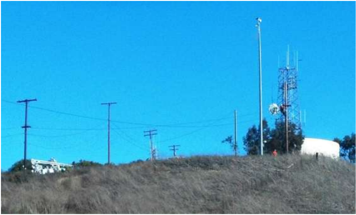
Figure 5: Pole installation/replacement and wire stringing on Segment 8, Phase 4.
