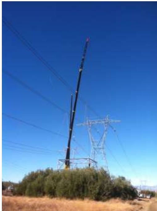
Figure 2: Segment 5 structure assembly occurring at Construct M90-T1X.
