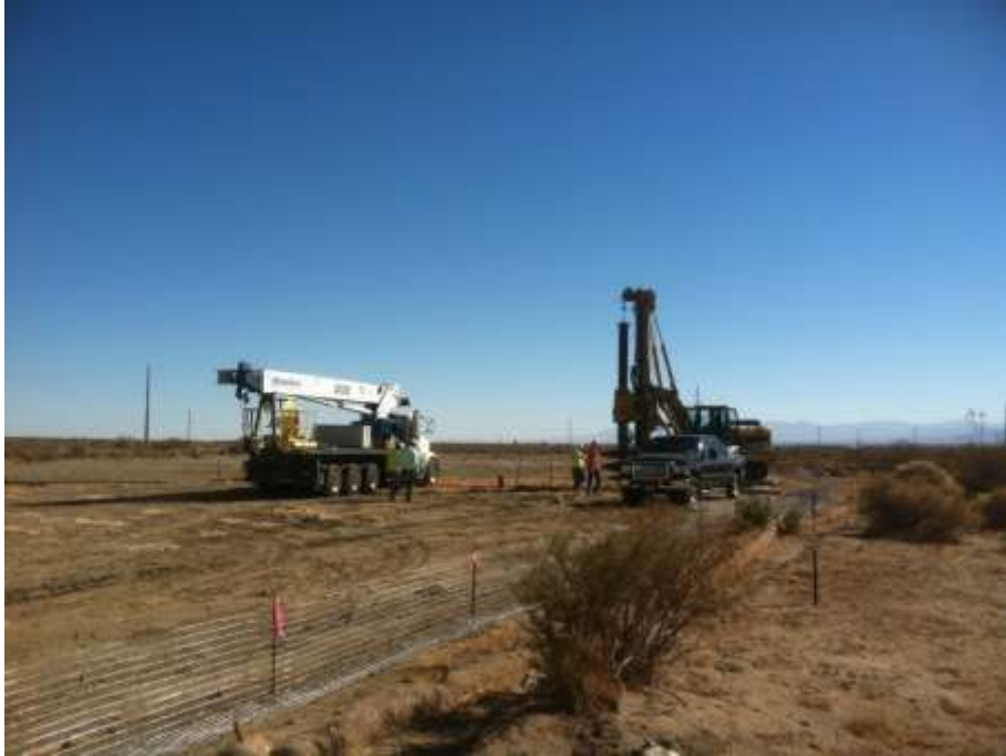
Figure 1: Segment 4 interset structure M74-T1X excavation.
