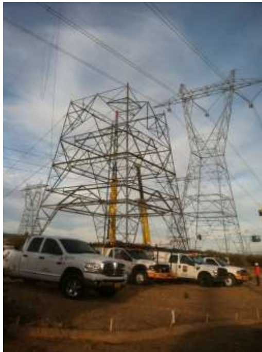
Figure 2: Segment 5 structure assembly occurring at Construct M90-T1X.
