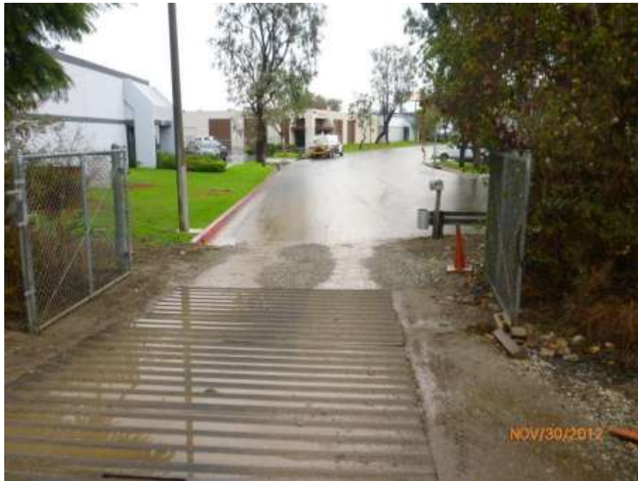
Figure 6: Sediment leaving the 605 contractor yard during a storm event.
