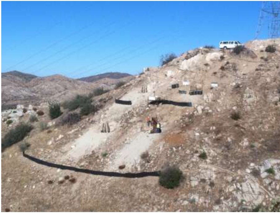
Figure 3: Segment 6 micropile pull tests occurring at Construct 18 (foundation activities).
