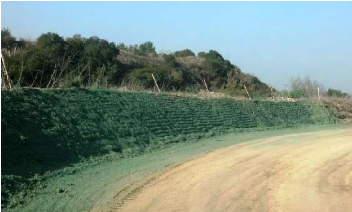
Figure 4: A cut slope hydroseeded for erosion control on Segment 8, Phase 4 in Rose Hills.
