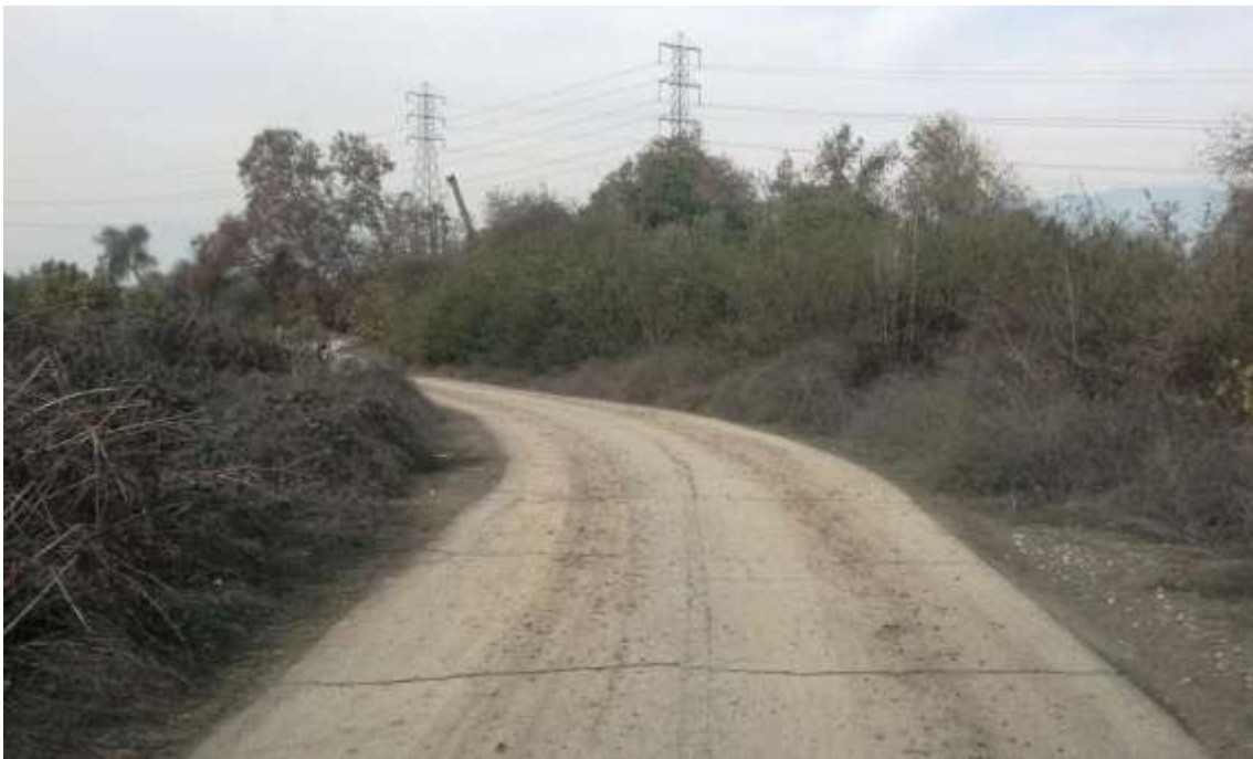
Figure 8: After rains early in the week, track out occurred on the access road to M42-T1. Crews used a sweeper truck and hand tools to clean the road throughout the day.
