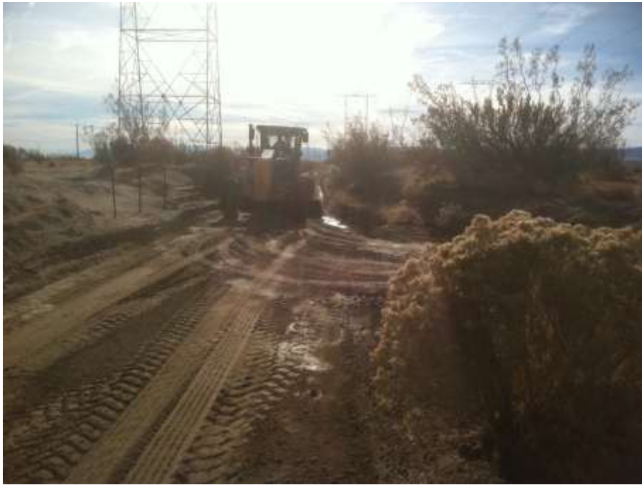
Figure 5: Segment 10 road grading activities south of Whirlwind Substation.
