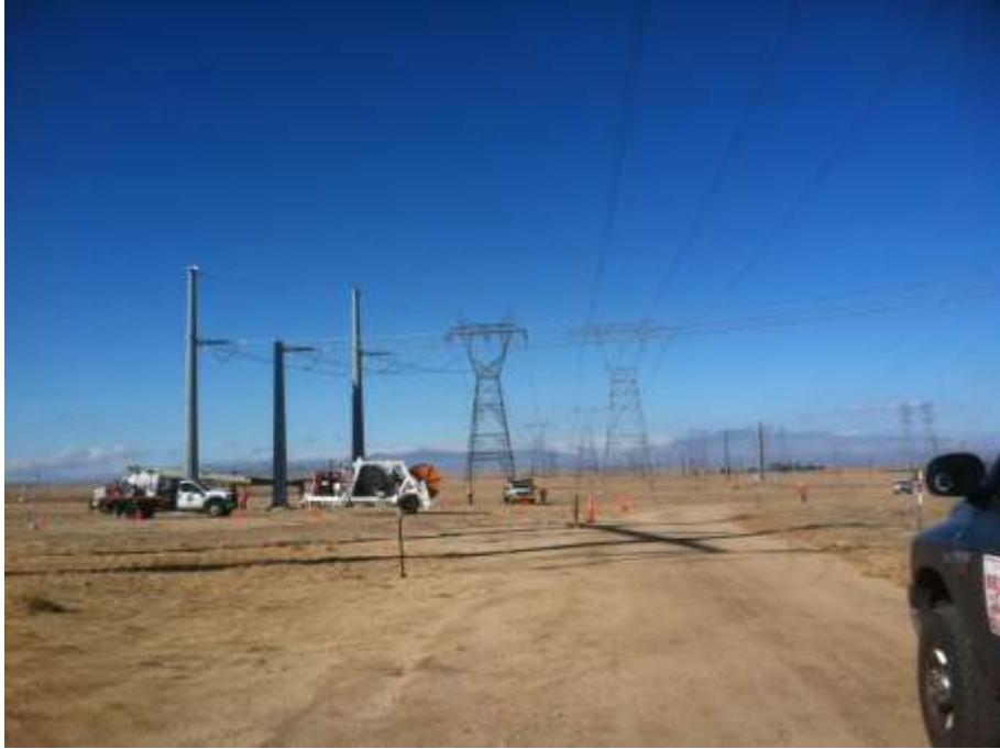
Figure 1: Segment 4 M25-T1 and M25-T2 wire and foundation removal activities.
