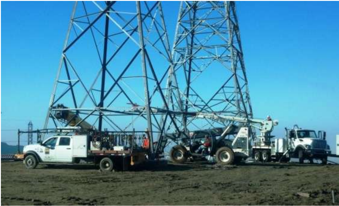
Figure 7: Wilson crews assemble towers at M45-T2, Segment 8, Phase 4.
