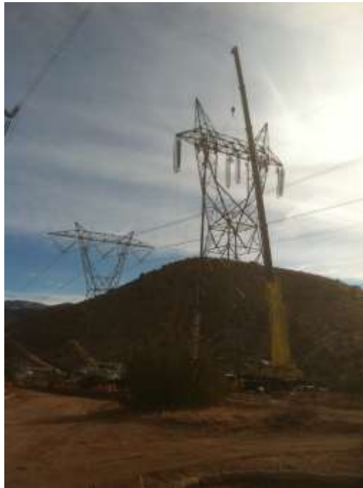
Figure 2: Segment 5 structure assembly occurring at Construct M111-T2X.
