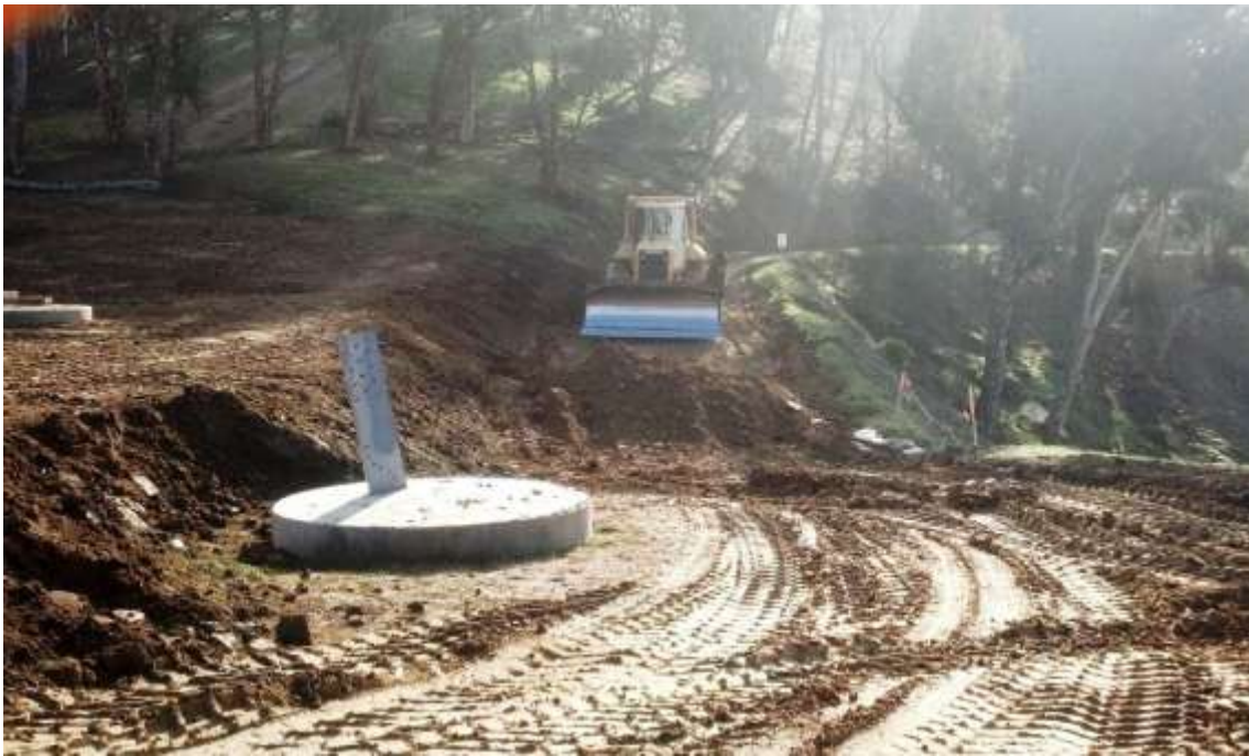
Figure 6: DCX performs road grading at M49-T3, Segment 8, Phase 4.
