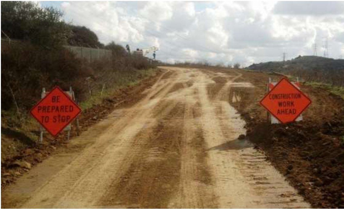
Figure 3: DCX crews installed signage at M45-T4, Segment 8, Phase 4..
