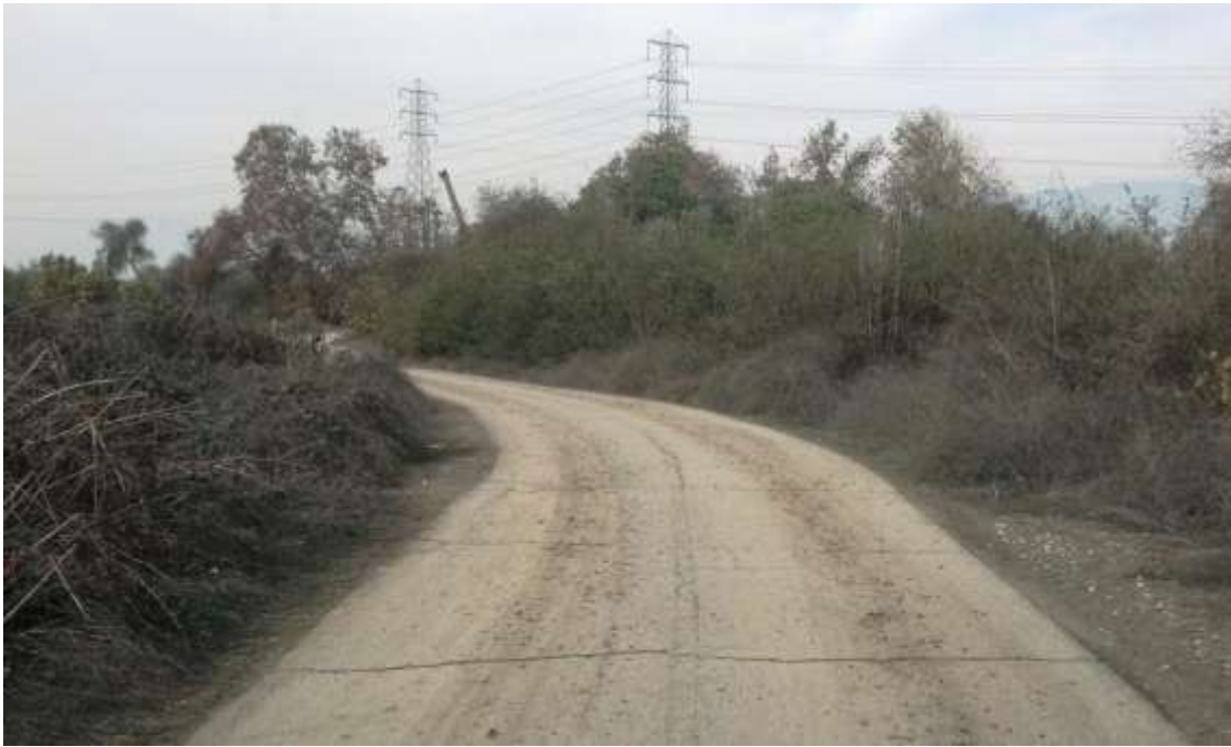
Figure 5: After rains early in the week, track out occurred on the access road to M42-T1. Crews used a sweeper truck and hand tools to clean the road throughout the day.
