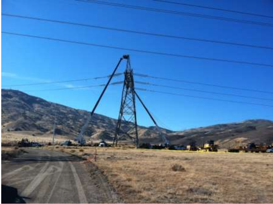
Figure 1: Segment 5, Construct 38 wire operations.
