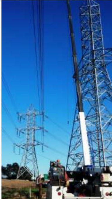
Figure 2: Tower assembly at M40-T4, Segment 8, Phase 4.
