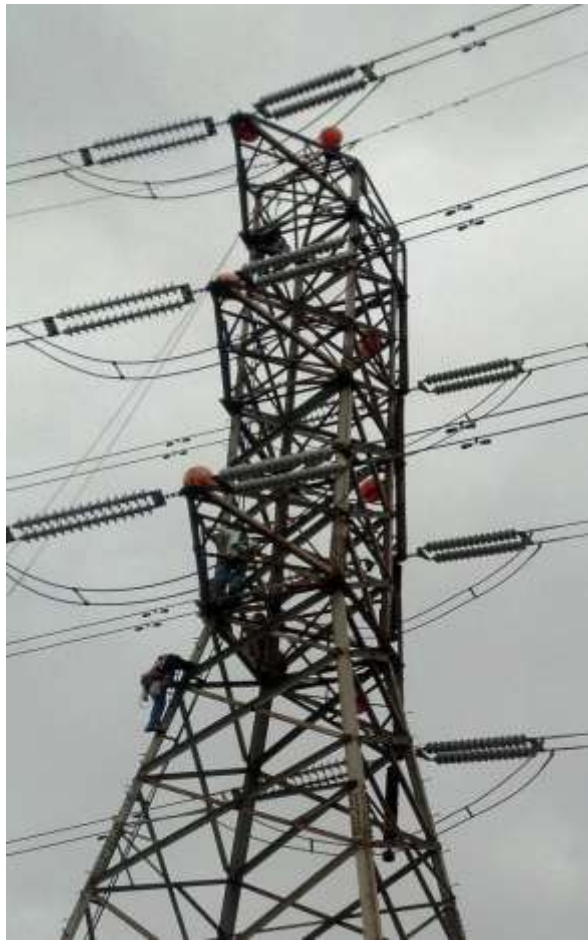
Figure 9: Nest deterrents installed in Construct M44-T2, Segment 8, Phase 4.
