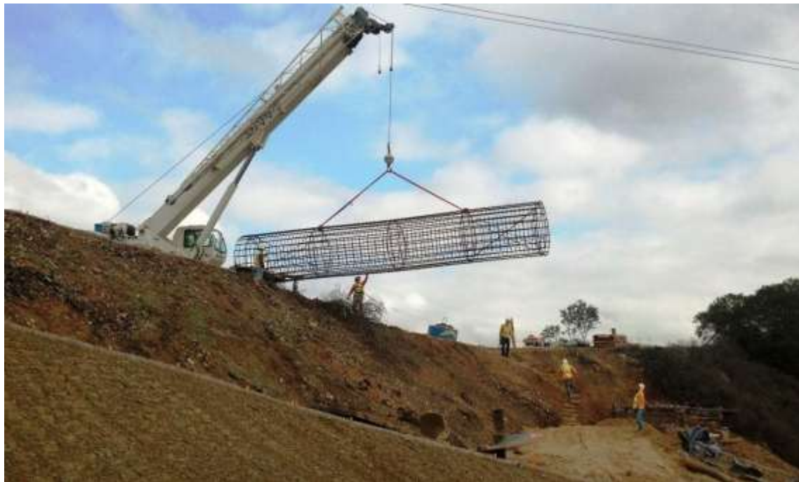
Figure 4: A DCX crew maneuvers a foundation cage at M45-T4, Segment 8, Phase 4.
