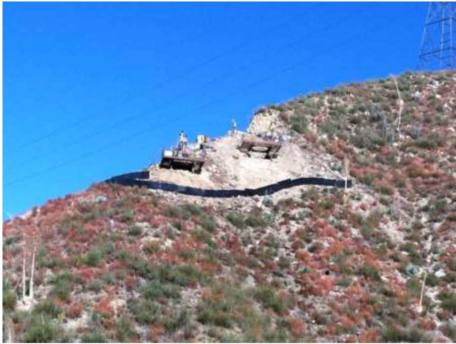
Figure 3: Micropile foundation installation occurring on Segment 6, Construct 60.
