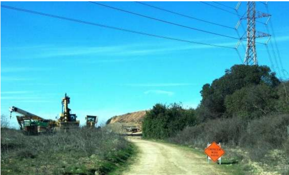
Figure 6: Sign informing the public of work occurring at M45-T4, Segment 8, Phase 4.
