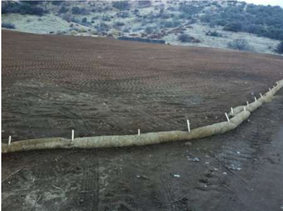
Figure 2: Hydroseeding application (BMPs) on Sagebrush Addendum Construct 236A wire stringing site.
