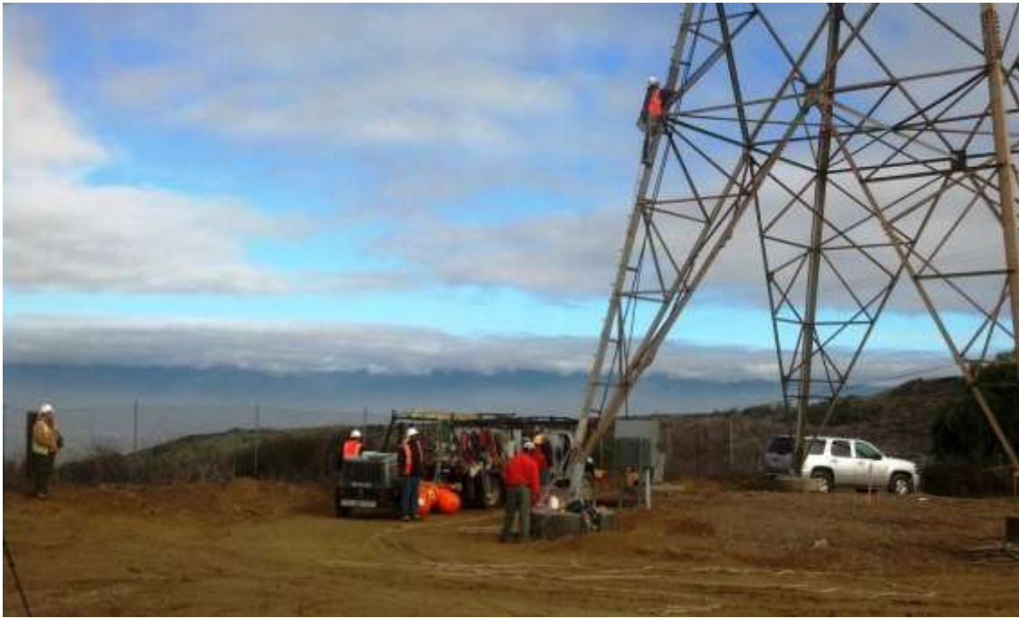
Figure 7: Linemen ascending Construct M44-T2, Segment 8, Phase 4 to perform nest removal.
