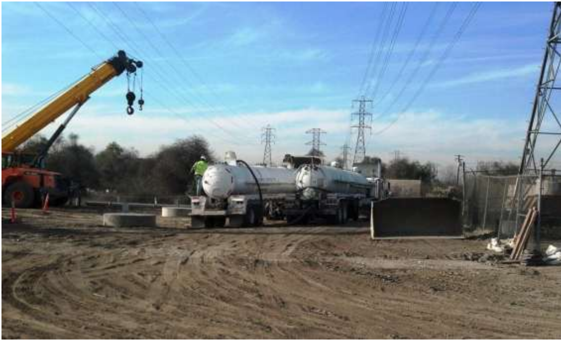
Figure 5: Crews pumping out Baker tanks at M42-T1, Segment 8, Phase 4.
