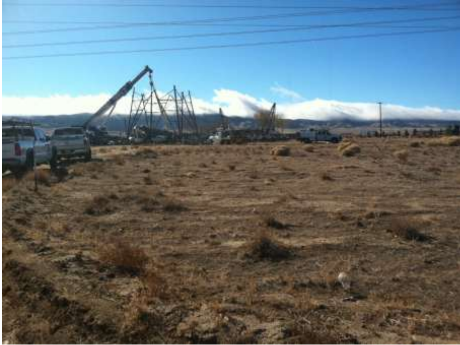
Figure 1: Segment 4, Construct M86-T2B erection operations.
