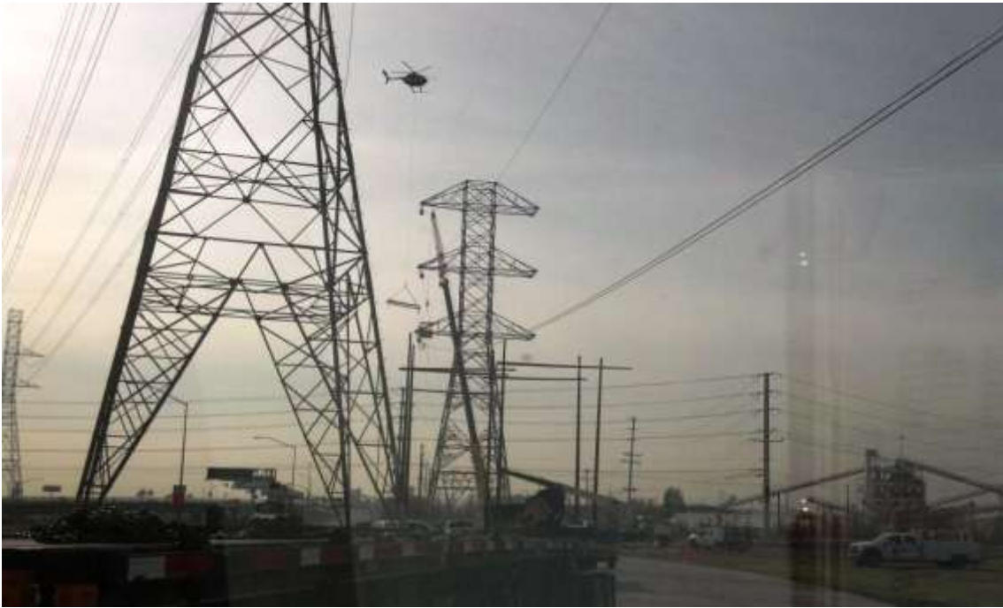
Figure 3: Wire stringing operations at Tower M31-T2, Segment 7.
