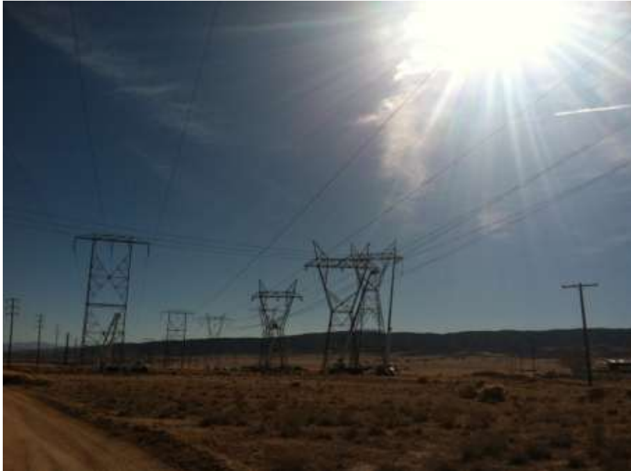
Figure 2: Segment 4, Wire stringing operations at Construct M86-T2A.
