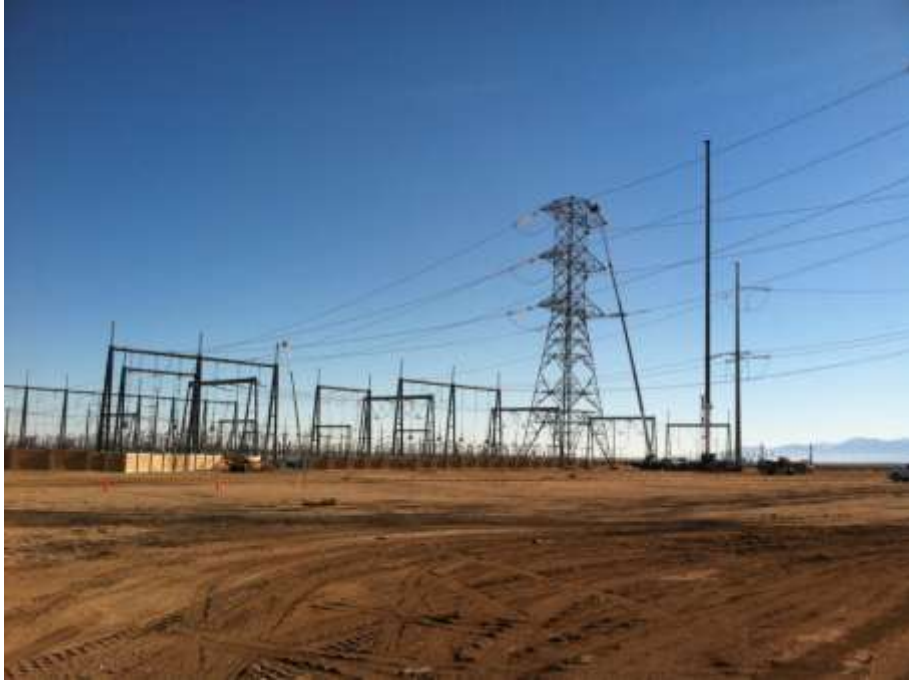
Figure 1: Segment 4, Wire stringing operations into Antelope Substation.
