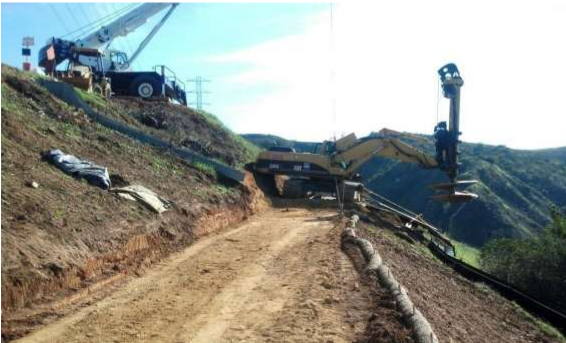
Figure 4: Foundation excavation at Tower M45-T5, Segment 8, Phase 4.
