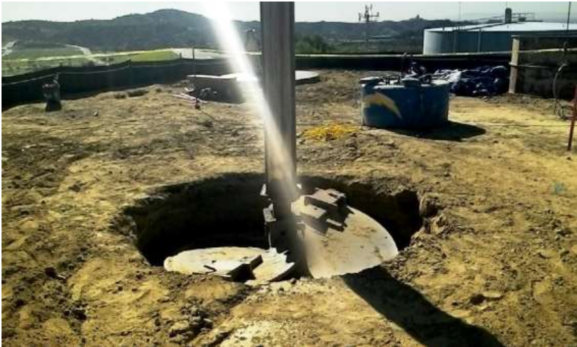
Figure 2: Foundation excavation/drilling at M44-T2, Segment 8, Phase 4.
