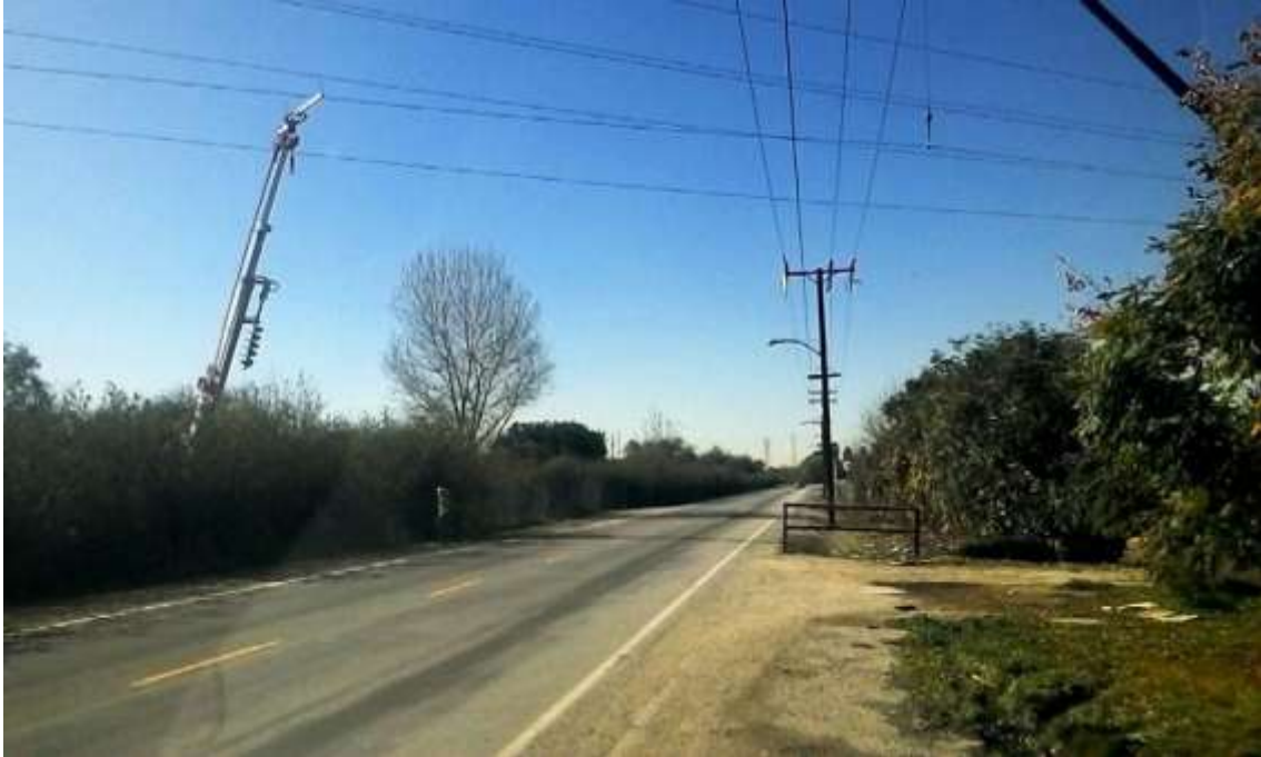
Figure 1: 66 kV wire stringing with guard structure across Durfee Road.
