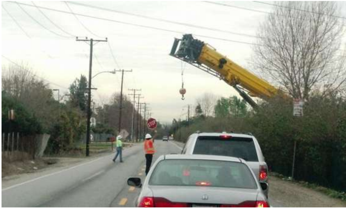
Figure 5: Traffic control on Durfee Road, Segment 8, Phase 4.
