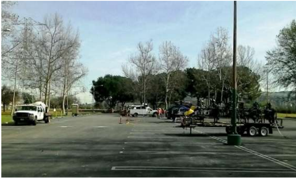
Figure 3: Wire stringing operations between Towers M38-T5 and M39-T4.
