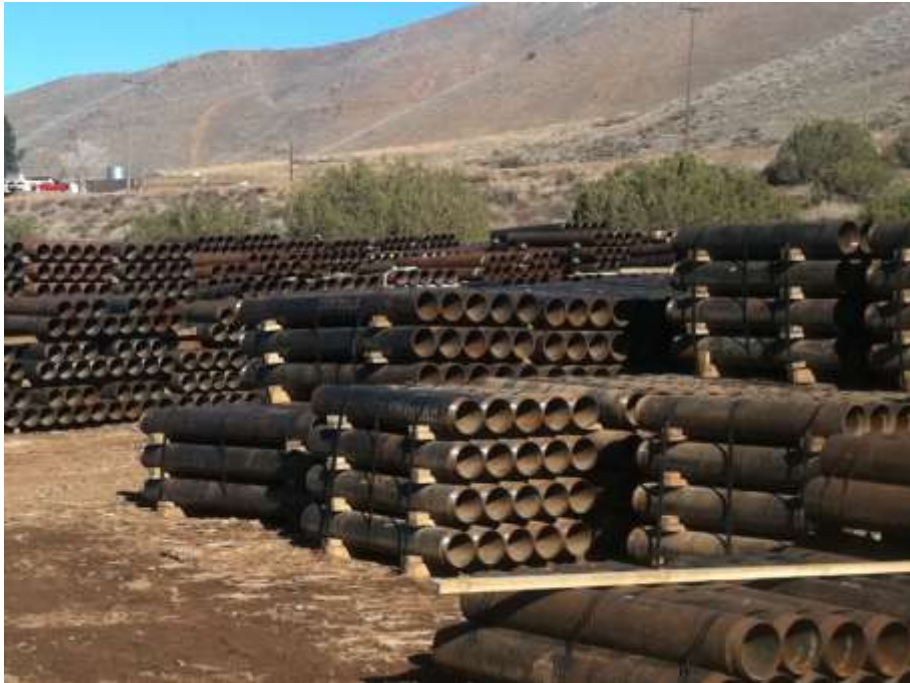
Figure 1: Micropile casings within the Vincent North Yard awaiting nest deterrent installation.
