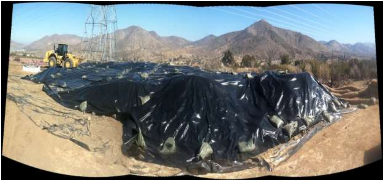
Figure 2: Construct 8 soil storage with visqueen covering during its storage.
