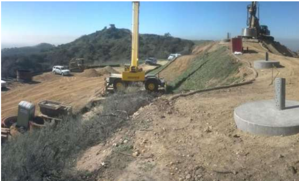
Figure 3: Foundation excavation at Tower M45-T4.
