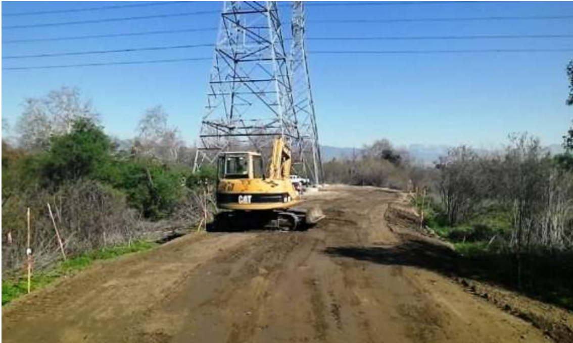
Figure 3: Road recontouring at the access road to Tower M42-T1A.
