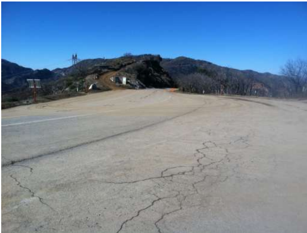
Figure 2: Trackout at Loop Road L and Angeles Forest Highway (Hwy 2).
