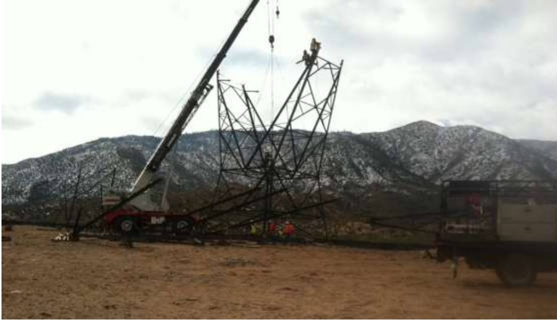
Figure 1: Tower erection at the Aliso HAY.
