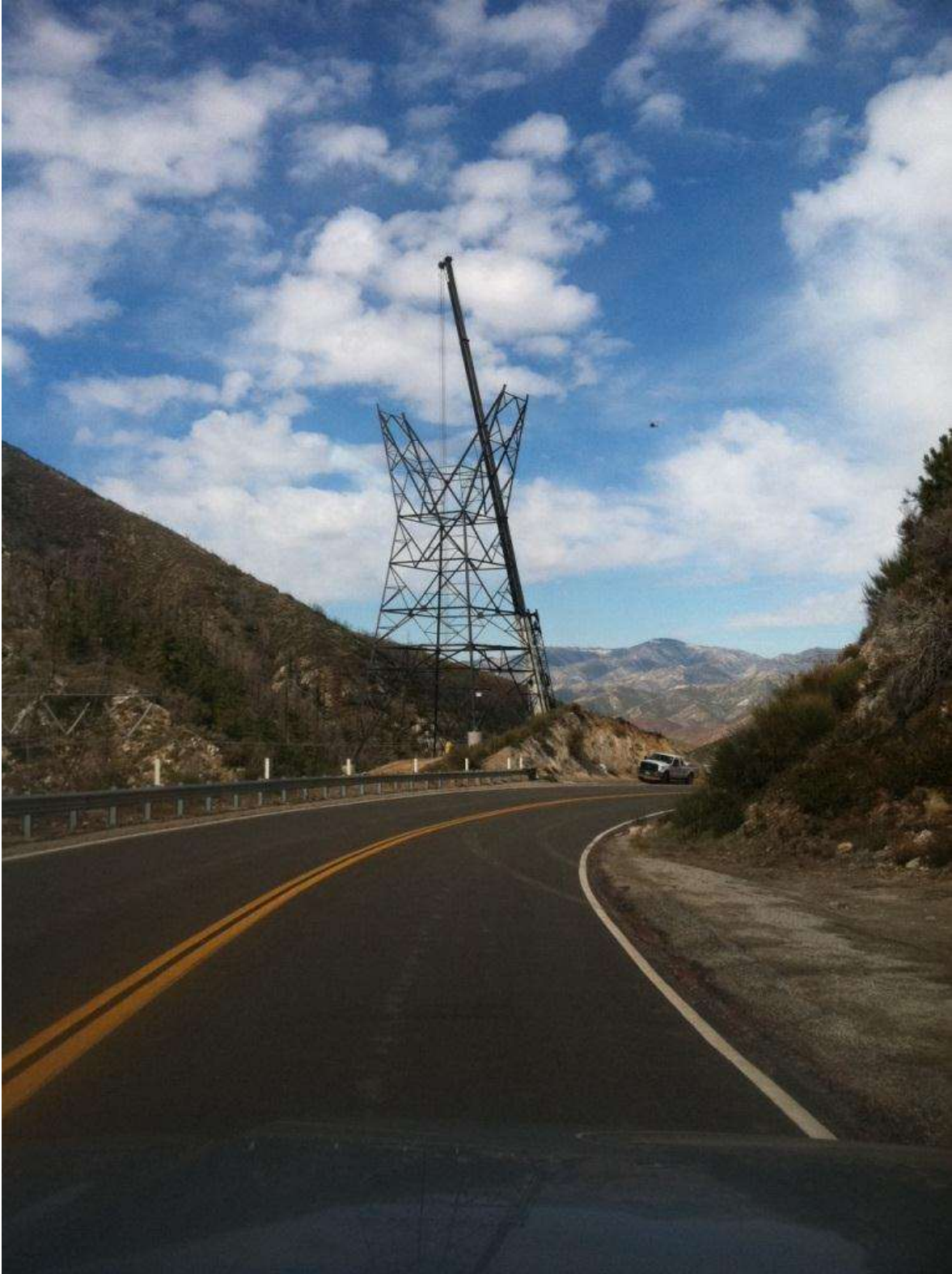
Figure 1: Structure erection at Construct 62.
