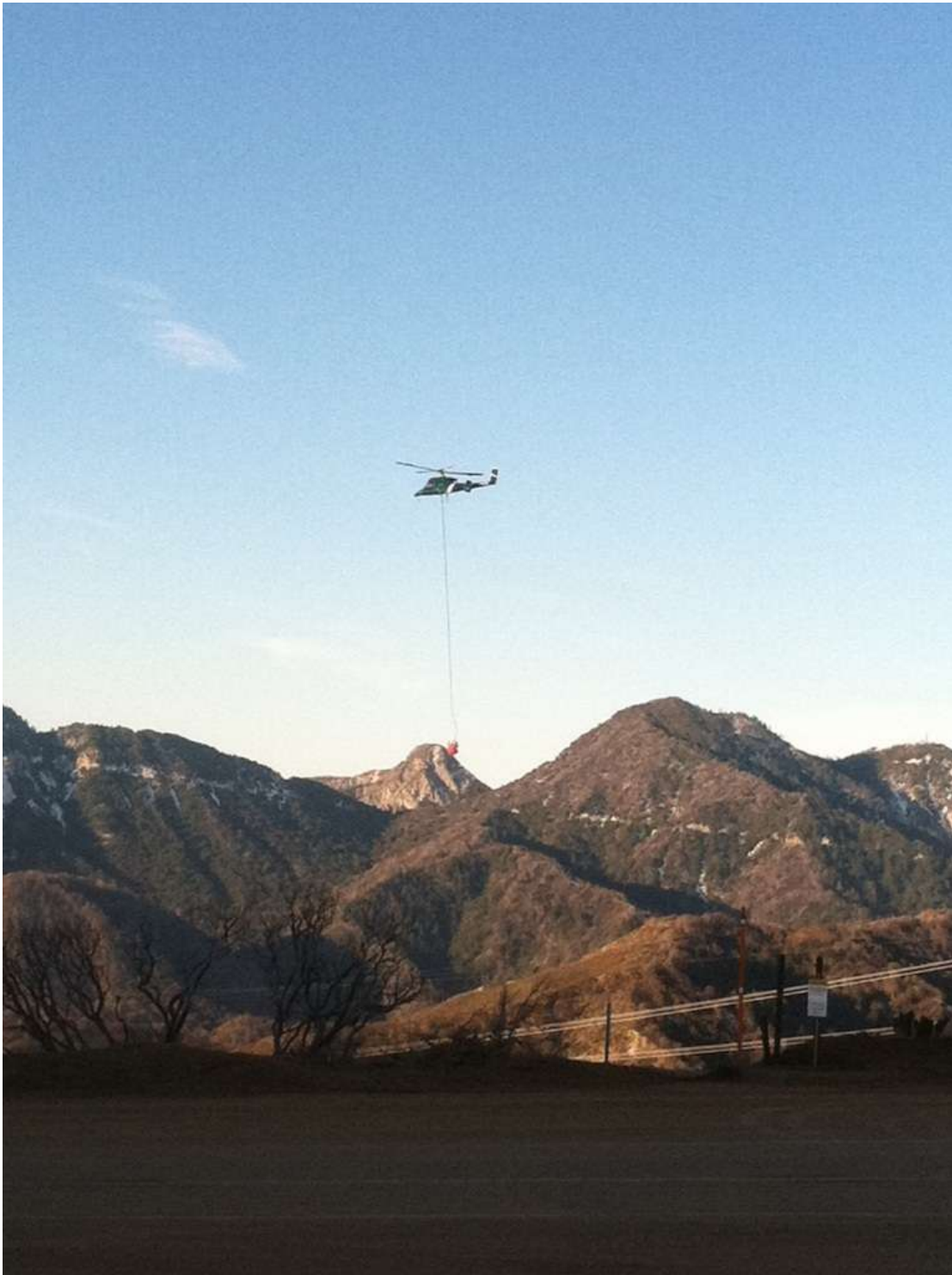
Figure 2: Dust control application via helicopter at Constructs along Loop Road L.
