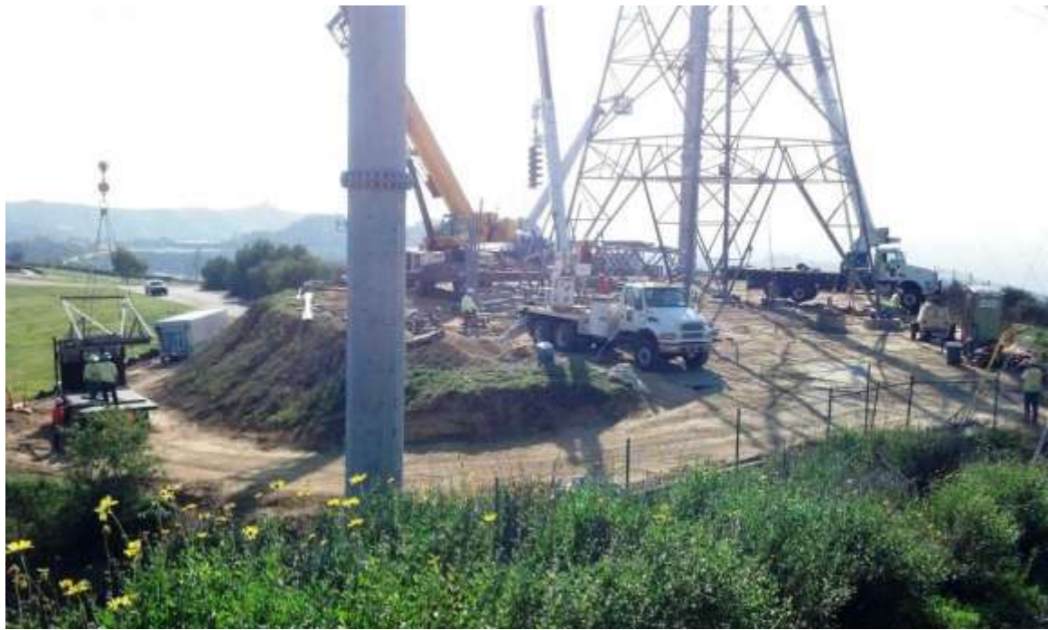
Figure 5: Tower work at the Rose Hills shoofly and M44-T2, Segment 8, Phase 4.
