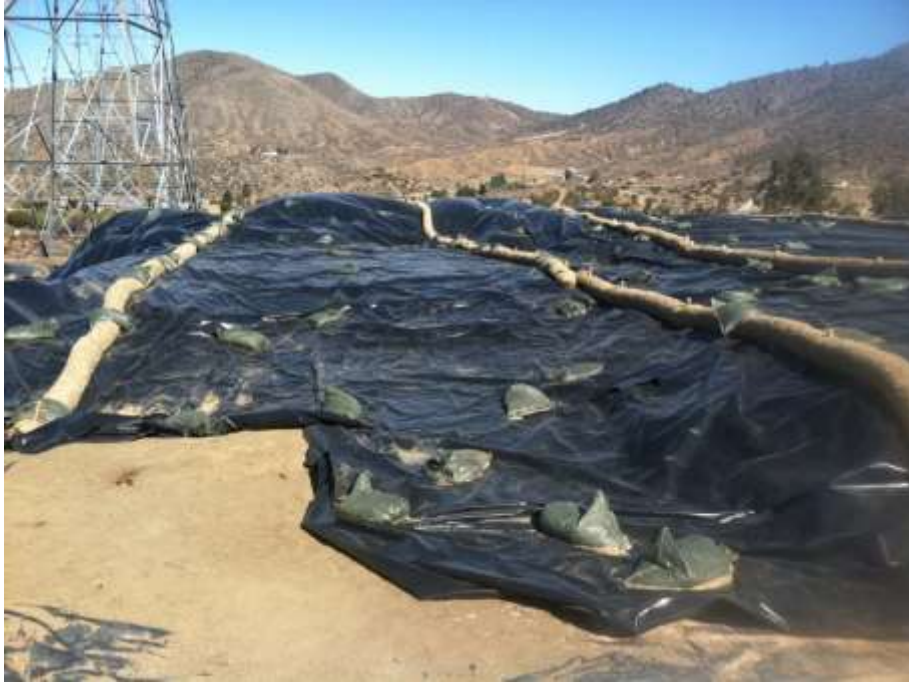
Figure 1: Soil storage at Construct 7 on Segment 6A.
