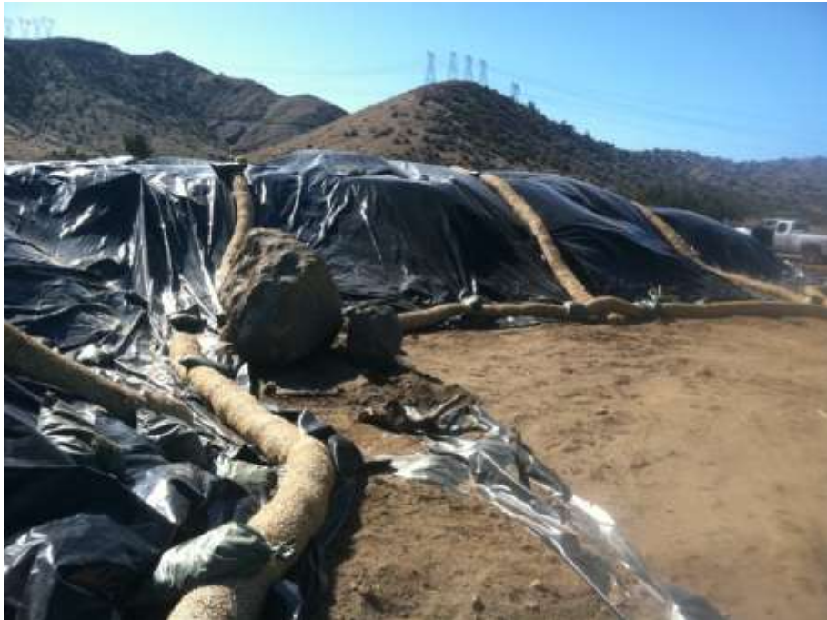
Figure 2: Soil storage at Construct 7 on Segment 6A.
