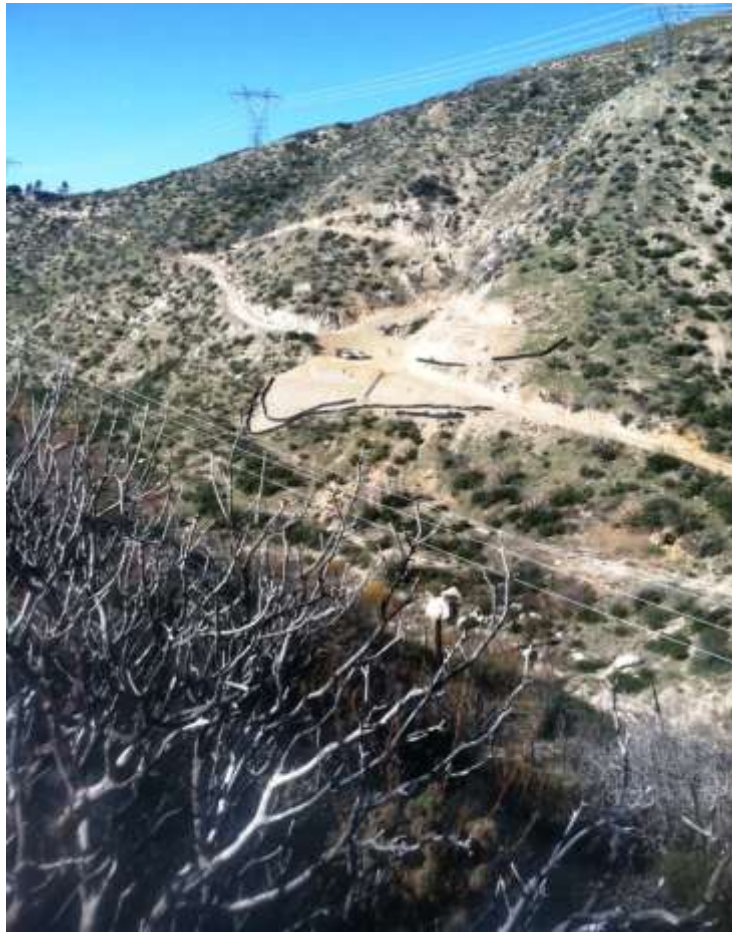
Figure 3: BMP installation at Construct 33 on Segment 6A.
