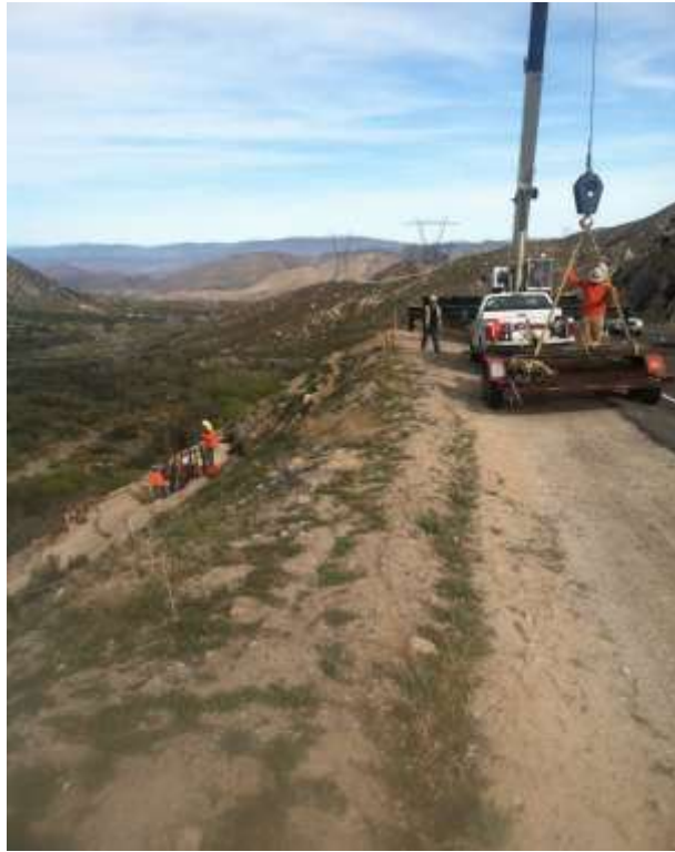
Figure 1: Foundation activities at Construct 28.
