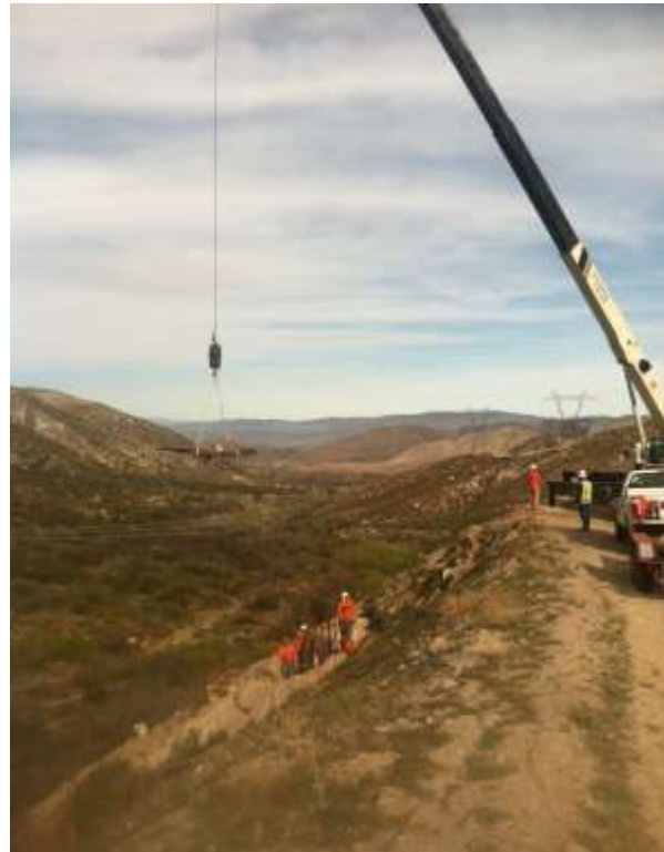
Figure 2: Foundation activities at Construct 28.
