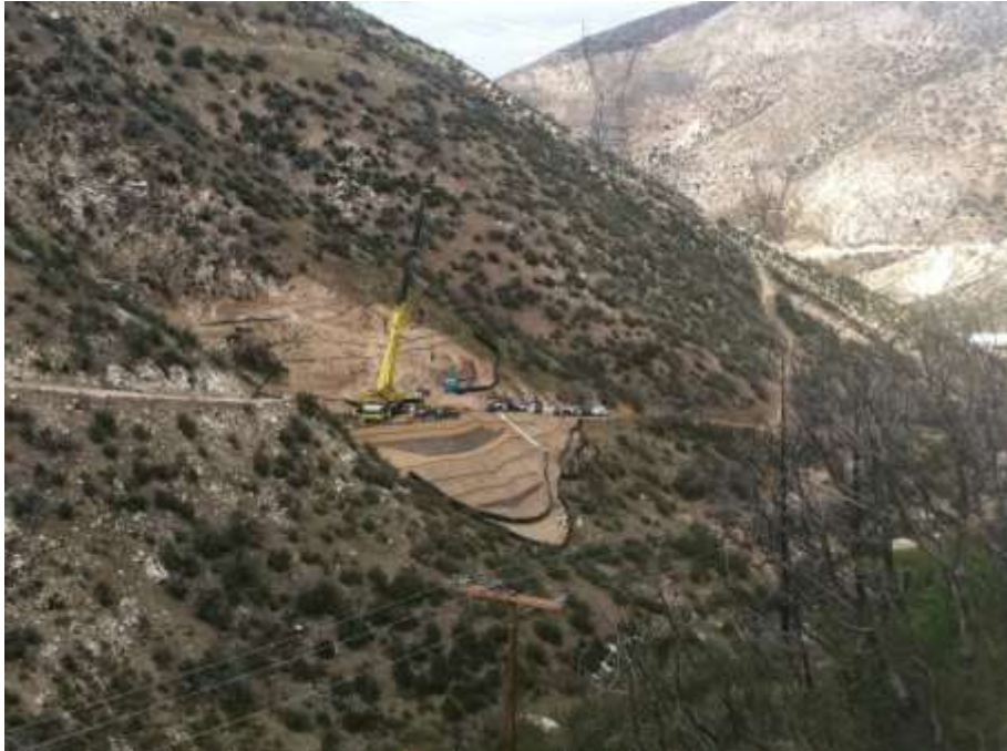
Figure 2: Structure assembly activities at Construct 33.
