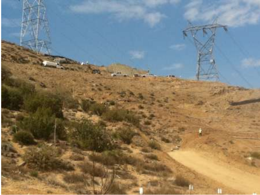
Figure 1: Grading activities at Construct 5.
