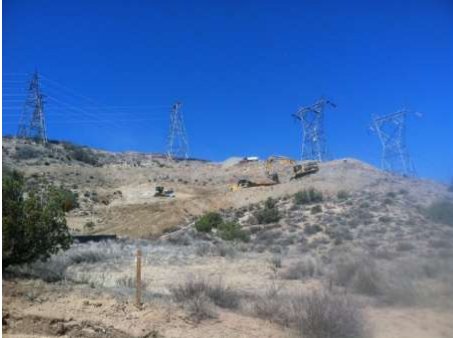
Figure 1: Grading activities at Construct 5.
