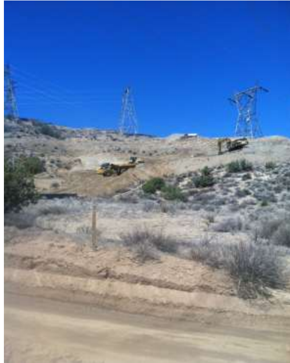
Figure 2: Grading activities at Construct 5.
