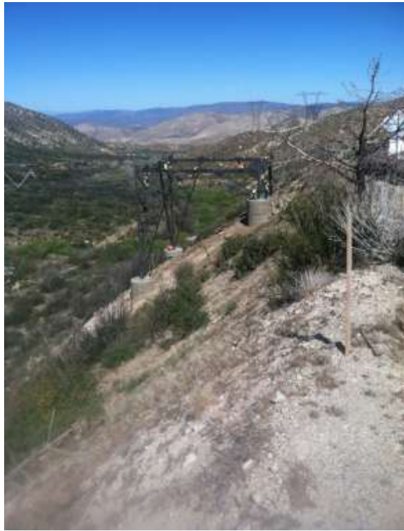
Figure 3: Erection activities at Construct 28.
