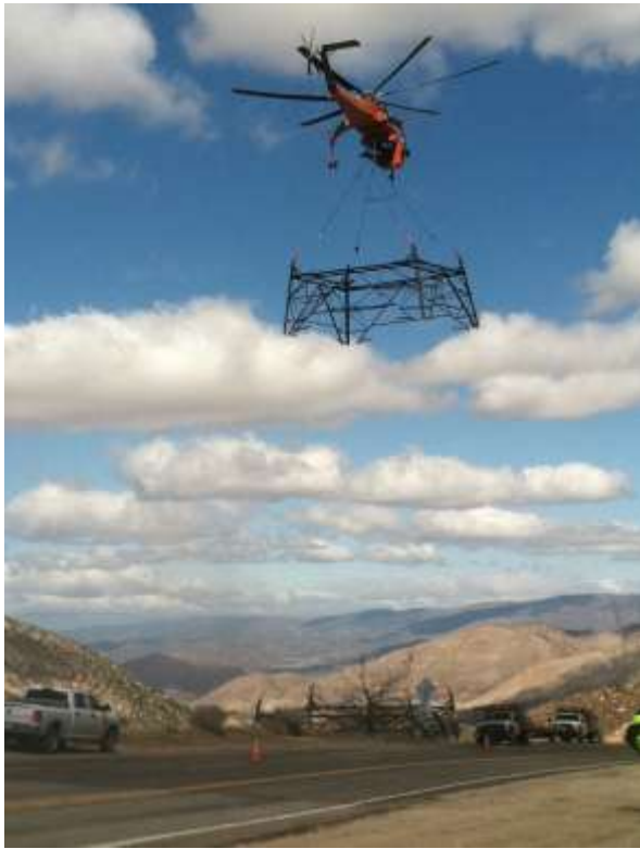
Figure 3: Erection activities at Construct 28.
