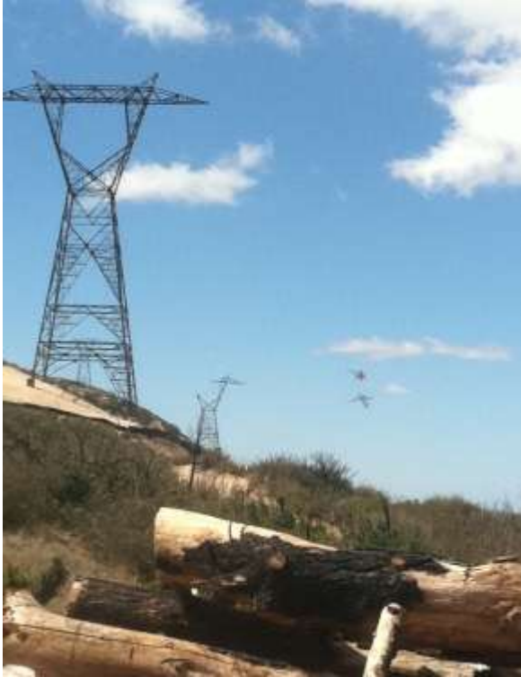
Figure 4: Erection activities at Construct 36.
