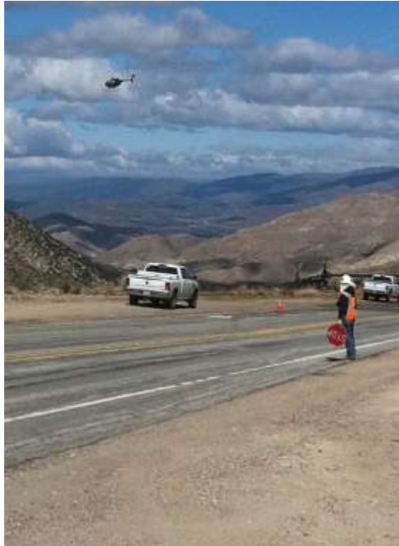
Figure 2: Aircrane erection activities occurring out of Aliso HAY to Construct 28.
