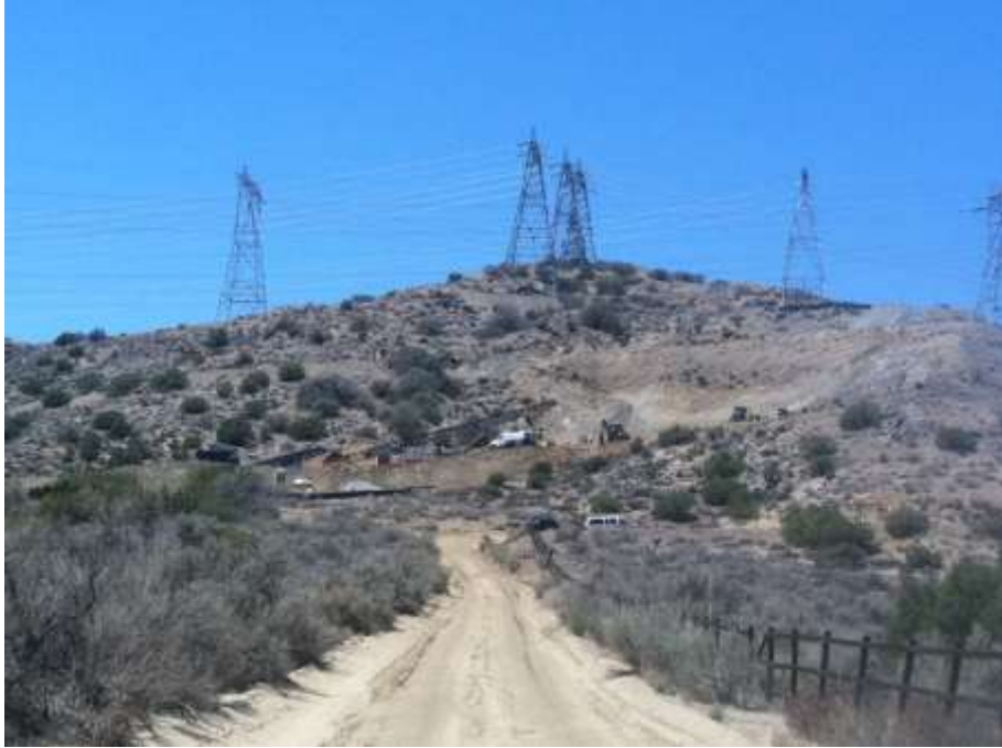
Figure 1: Tower site grading activities at Construct 5, Segment 6.
