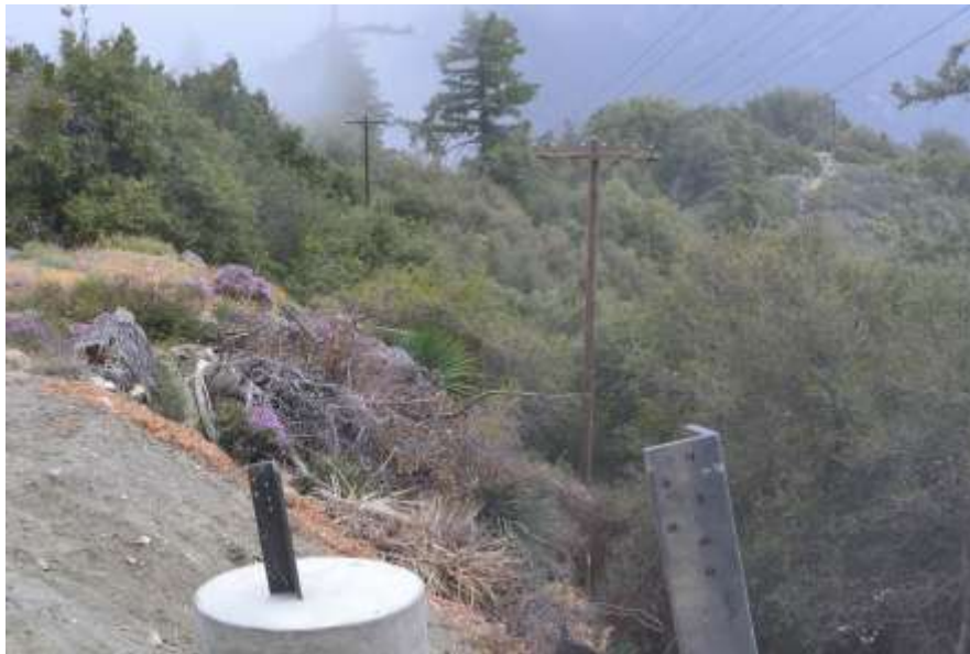
Figure 4: Telecom line proposed for removal near Tower 95 in Segment 6C.
