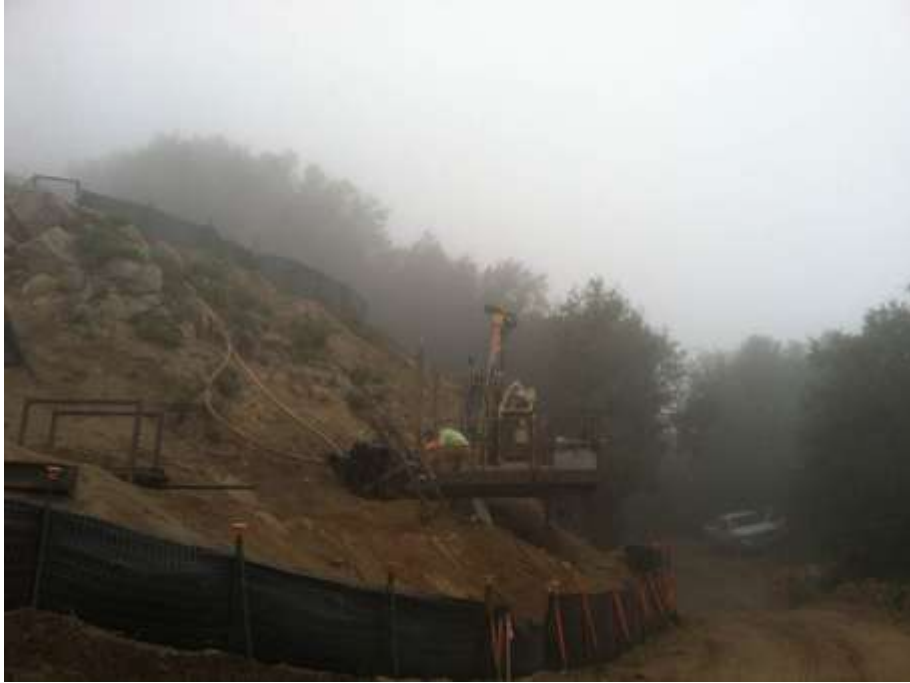
Figure 1: Foundation installation by micropile crews at Tower 100, Segment 6C.
