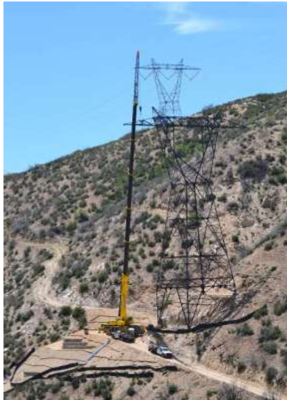
Figure 2: Erection of Tower 33, Segment 6A.
