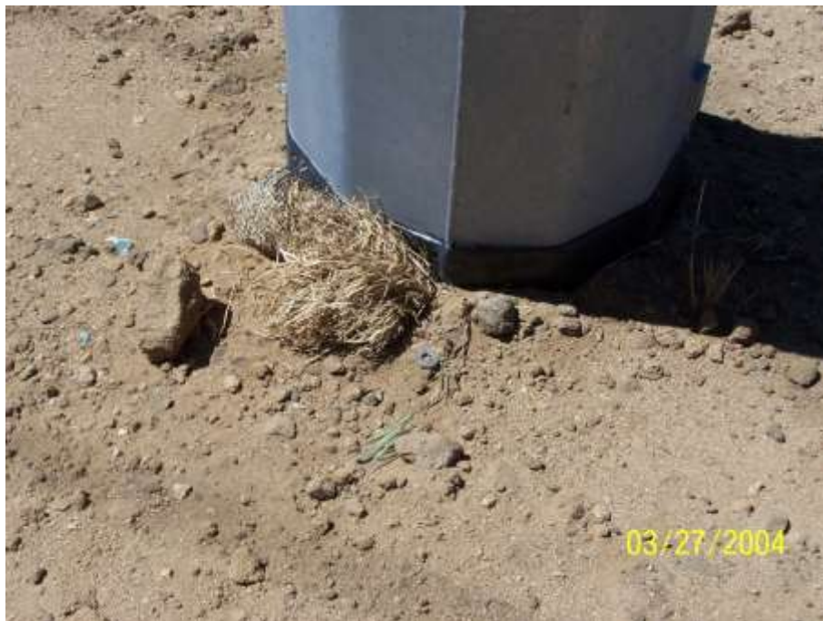
Figure 2: Segment 3B microtrash noted at Construct 34.
