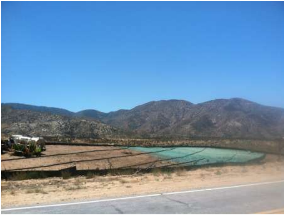
Figure 3: Hydromulching application (BMP installation) at Aliso HAY.
