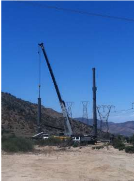
Figure 1: Structure assembly at Construct 11 on Segment 6A.
