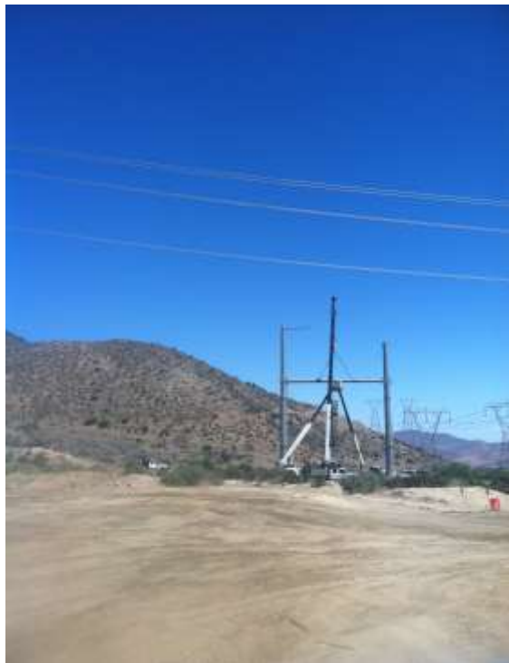
Figure 2: Structure assembly at Construct 11 on Segment 6A.
