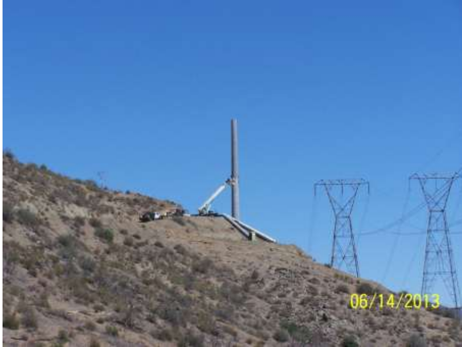
Figure 1: Structure assembly at Construct 10 on Segment 6A.
