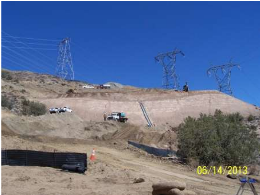
Figure 2: Grading activities at Construct 5 on Segment 6A.
