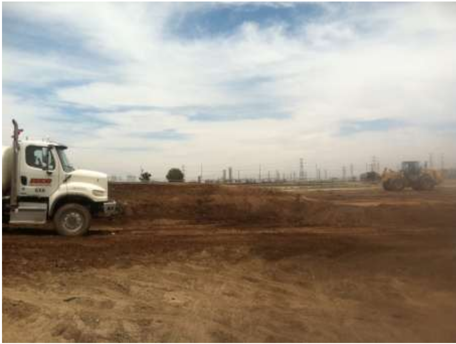
Figure 3: Grading activities at Tower M72-T5 on Segment 8, Phase 3.
