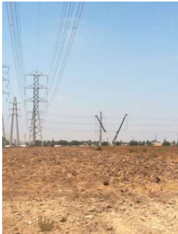
Figure 2: Foundation activities at Tower M73-T1, Segment 8, Phase 3.
