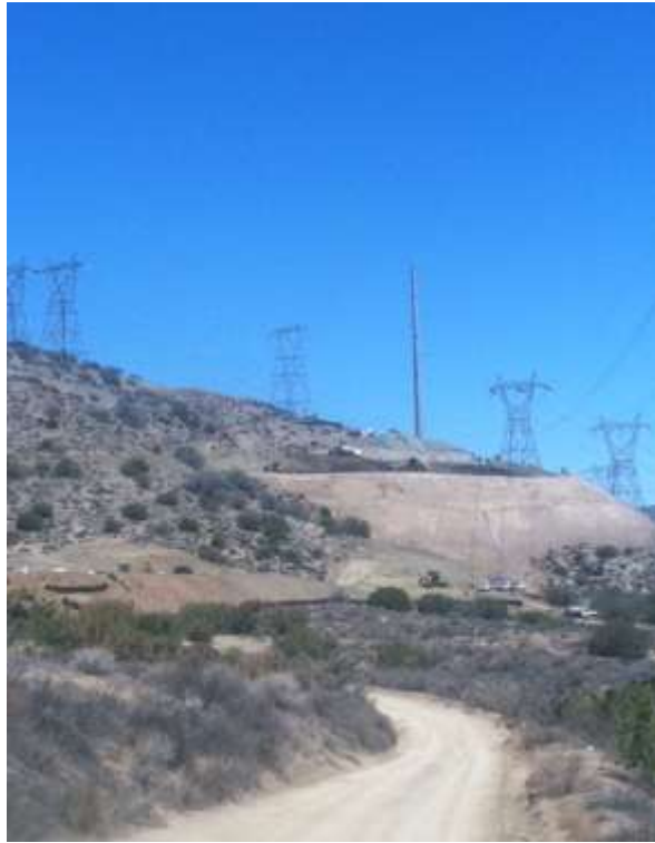
Figure 1: Grading activities at Construct 5, Segment 6A.
