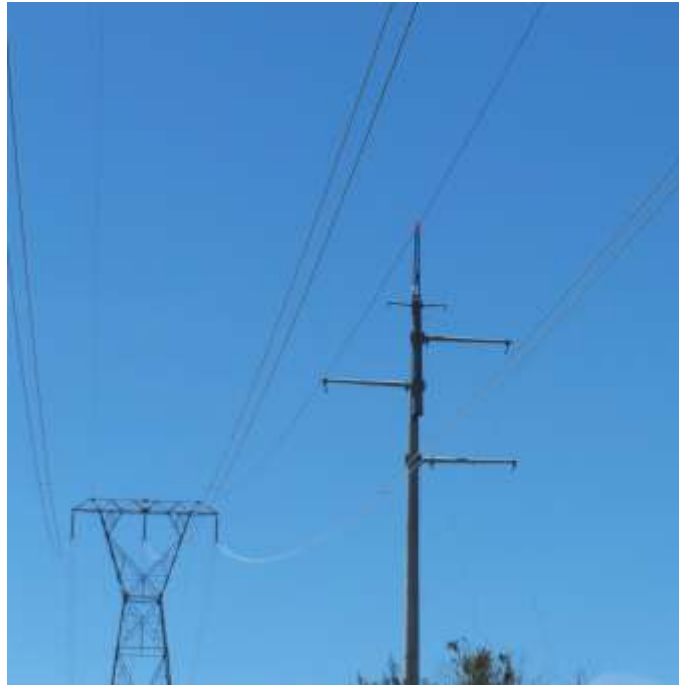
Figure 1: Structure assembly at Construct 14 on Segment 6.
