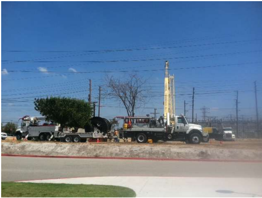
Figure 3: Cable pulling activities at Vault 43218 on Segment 8 66 kV.
