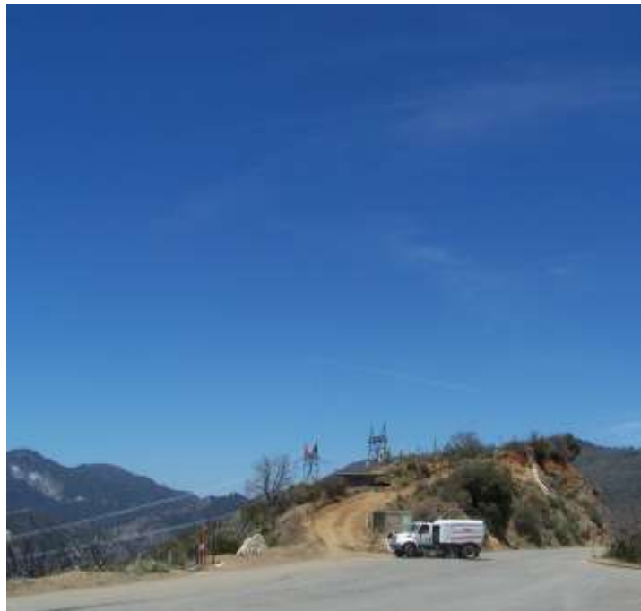
Figure 2: Fugitive dust control at Angeles Crest Highway on Segment 6.
