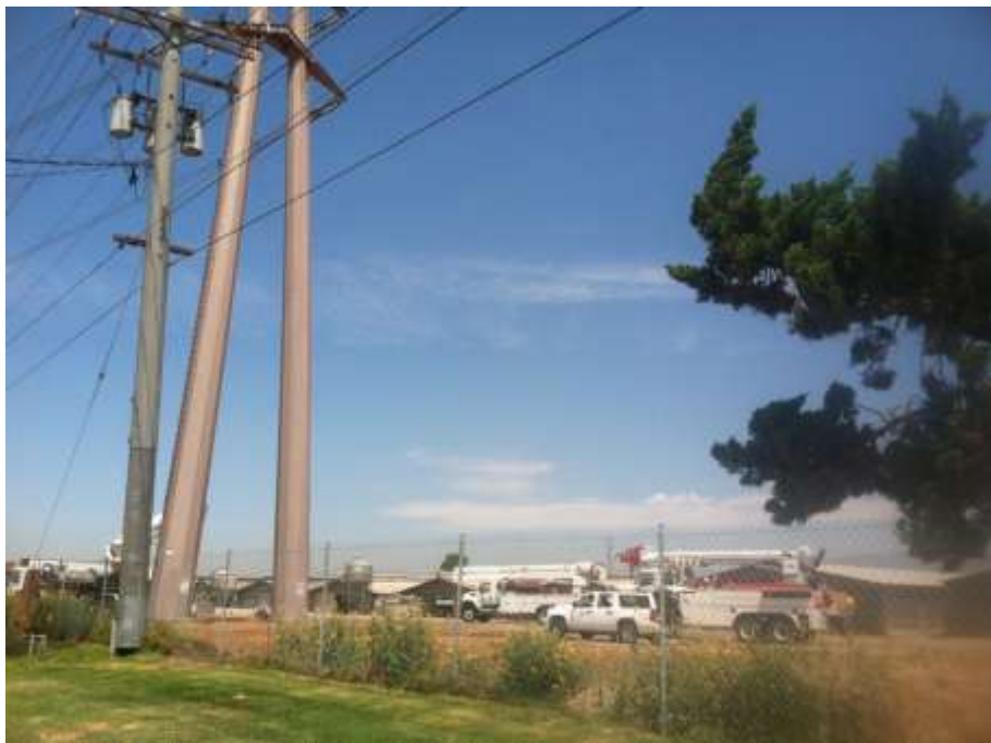
Figure 2: Wire removal preparation on Segment 8, Phase 3, Tower M2-T5.
