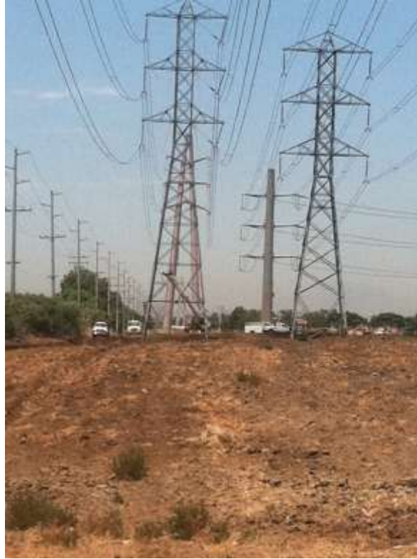
Figure 1: Foundation installation on Segment 8, Phase 3, Tower M73-T3.
