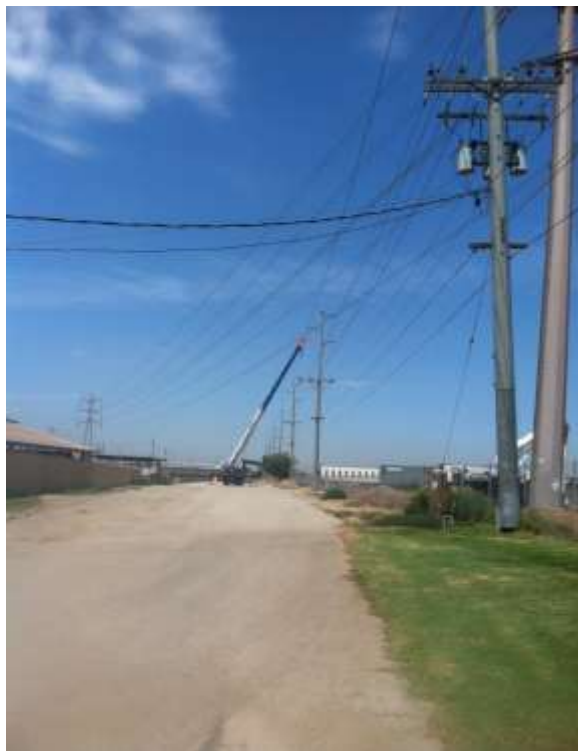
Figure 2: Wire removal preparation on Segment 8, Phase 3, Tower M2-T5.
