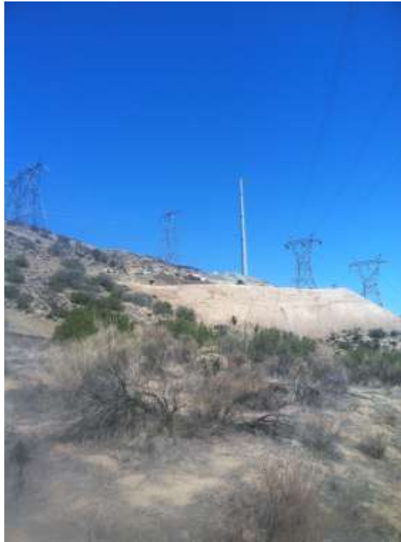
Figure 1: Grading activities occurring on Segment 6A Construct 5.
