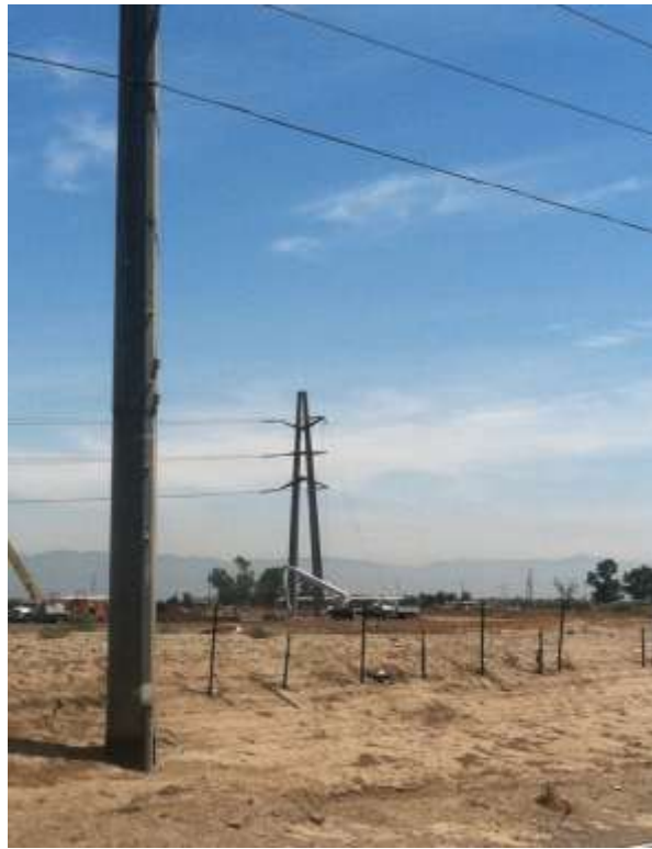
Figure 3: Wire removal activities on Segment 8, Phase 3, Tower M1-T4.
