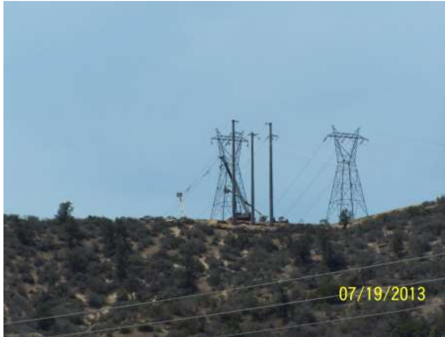
Figure 1: Structure erection and wire relocation activities at Construct 19 on Segment 6.
