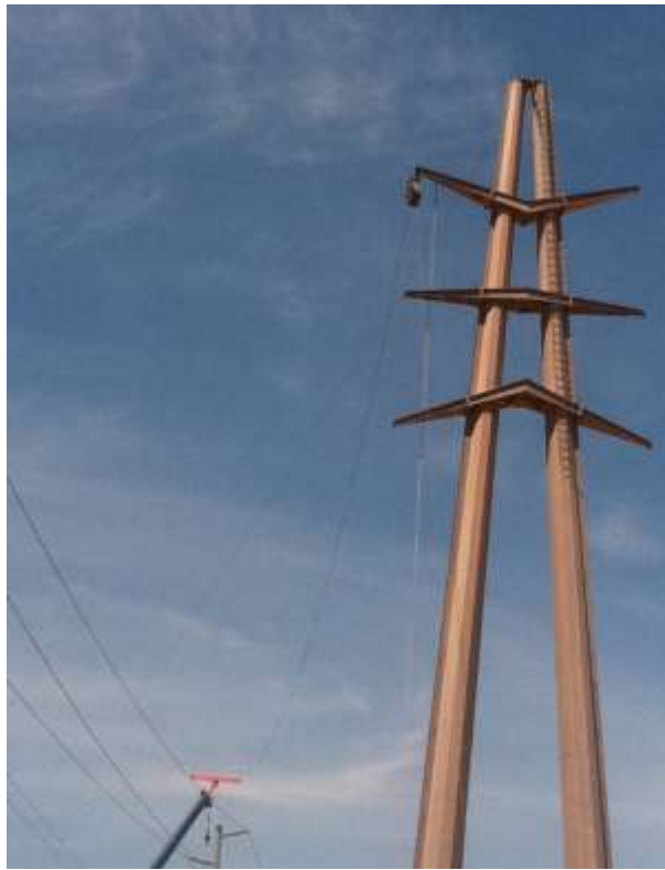
Figure 4: Wire removal activities on Segment 8, Phase 3, Tower M2-T5.
