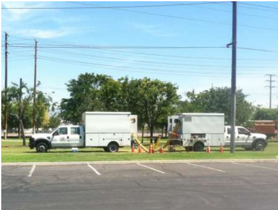
Figure 2: 66 kV activities at Vault 43213 on Segment 8.
