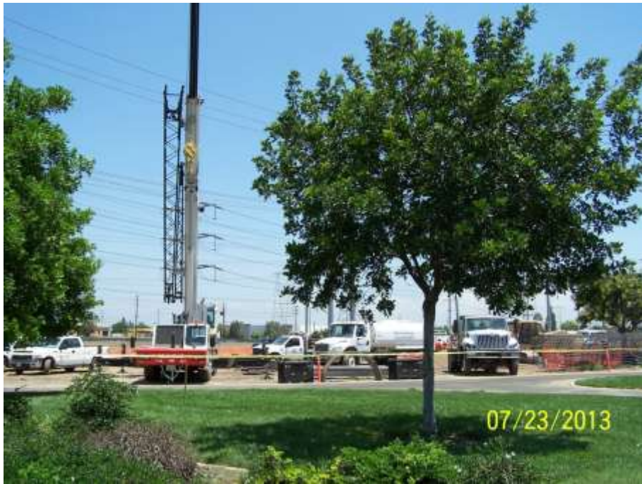
Figure 3: Foundation activities at Tower M66-T8/J8, Segment 8, Phase 3.
