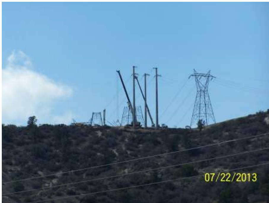
Figure 2: Wire transfer at Construct 19, Segment 6.
