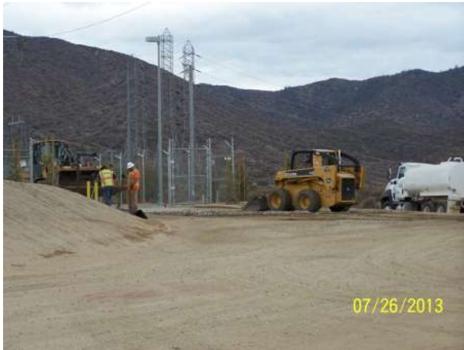
Figure 1: Stabilized Construction Entry installation at Vincent Substation, Segment 9.
