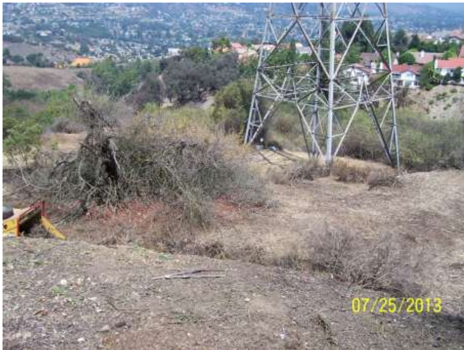
Figure 4: Vegetation removal activities on Tower 49-2, Segment 8, Phase 4.
