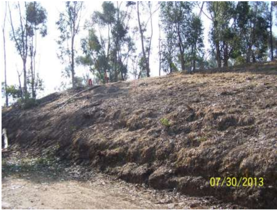
Figure 3: Vegetation clearing at Tower M49-T2 on Segment 8, Phase 4.
