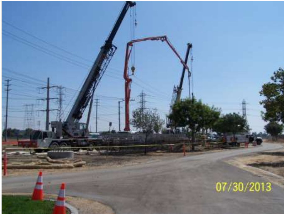
Figure 2: Foundation activities at Tower M66-T8, Segment 8, Phase 3.
