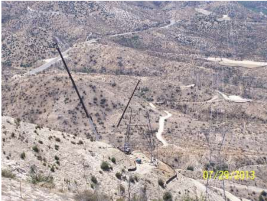
Figure 1: Segment 6 Construct 20 tower erection activities.
