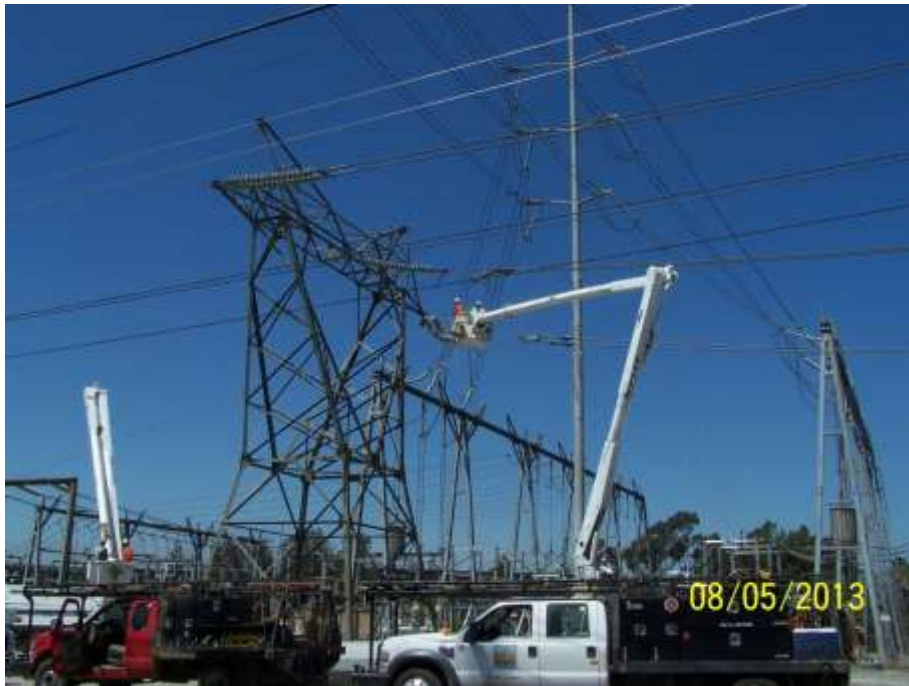
Figure 2: Segment 11B Construct 72(M8-T4) wire stringing removal and wreckout.
