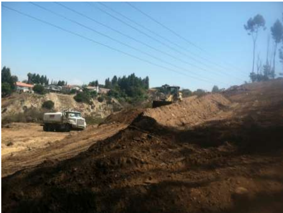
Figure 4: Grading activities occurred at Tower M49-T2 on Segment 8, Phase 4.
