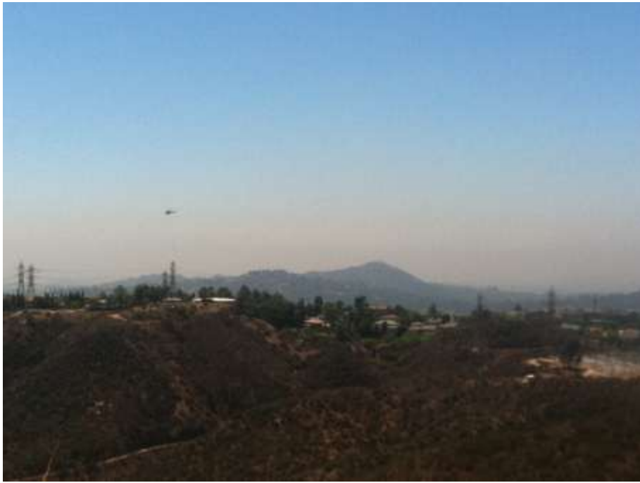
Figure 3: Wire stringing operations occurred near Gould Substation on Segment 11B.
