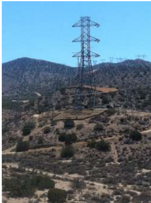
Figure 2: Wire stringing activities occurred at Construct 2 on Segment 6.
