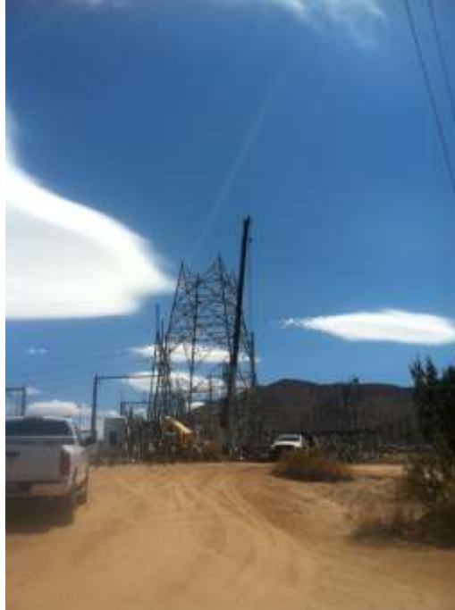
Figure 1: Assembly activities occurring at Construct 1 on Segment 6.
