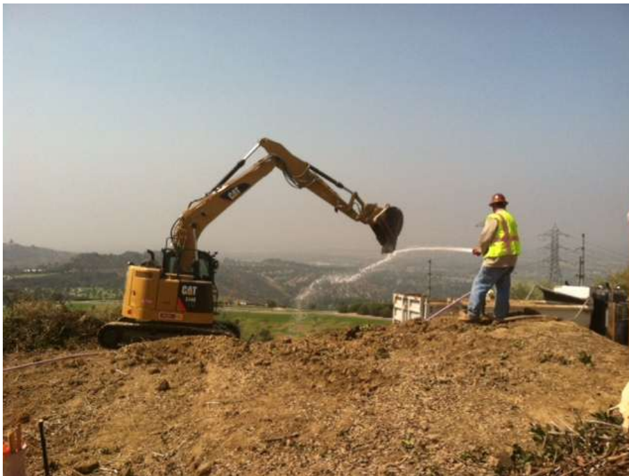
Figure 6: Road grading at Segment 8, Tower M44-T3.
