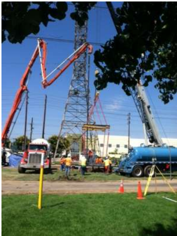
Figure 5: Concrete pouring activities on Segment 8, Tower M32-T6.
