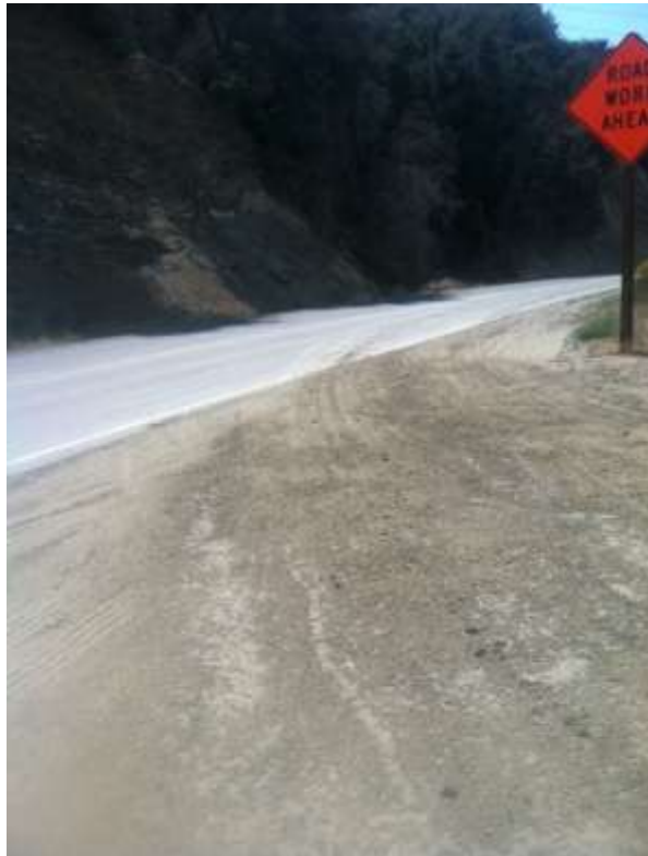
Figure 3: Trackout observed from Loop Road L along Upper Big Tujunga on Segment 6.
