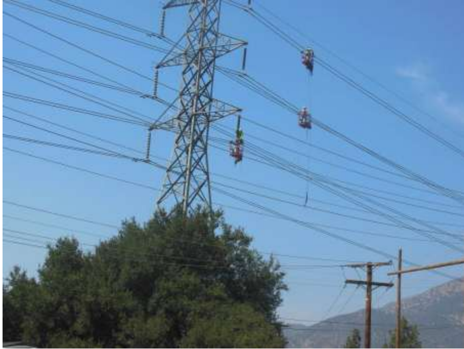
Figure 1: Hanging spacers on completed wire string along Segment 11B.
