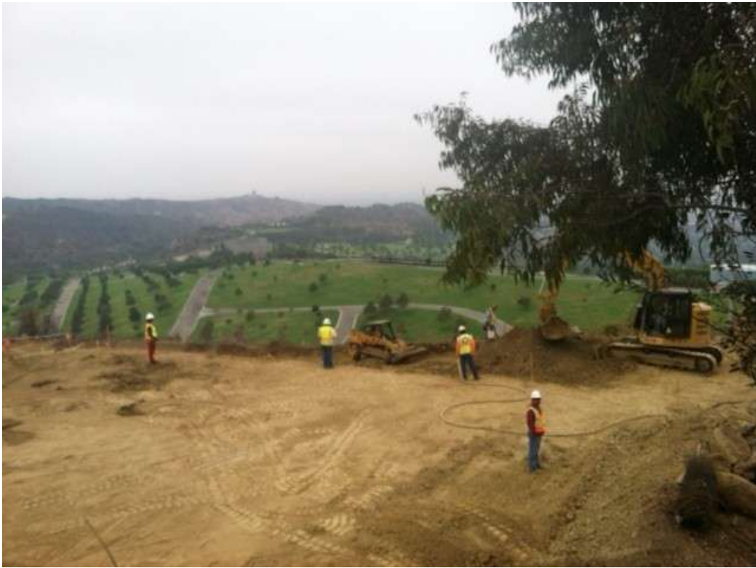
Figure 7: Road grading activities at Segment 8, Tower M44-T3.
