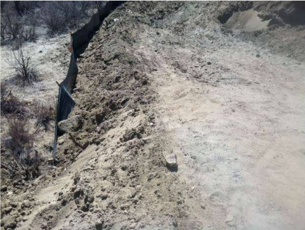
Figure 4: Silt fence buried east of the Construct 4 foundation at Segment 6.
