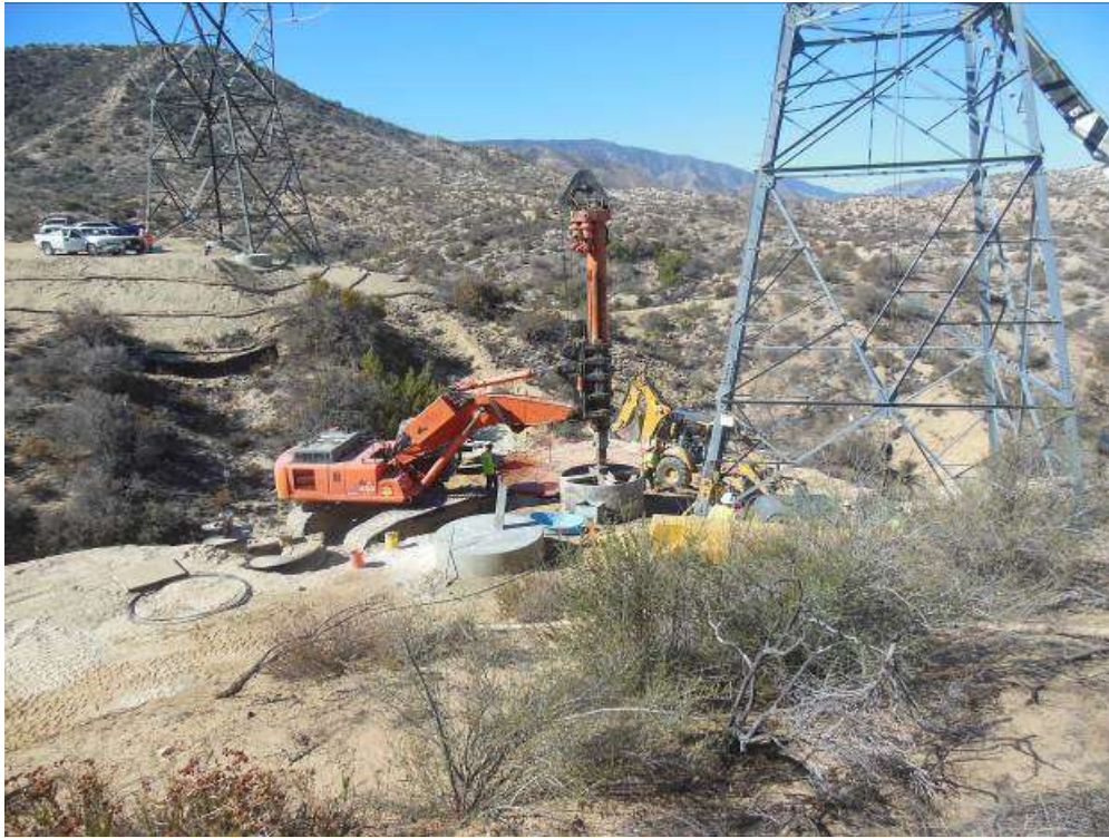
Figure 1: Foundation excavation at Construct 17 along Segment 6.
