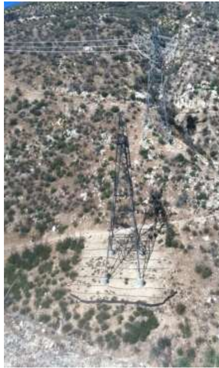
Figure 1: Wire stringing operation at Construct 32 on Segment 6.
