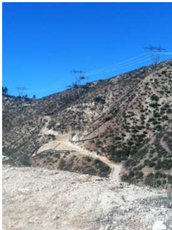
Figure 2: Wire stringing at Construct 33 on Segment 6.
