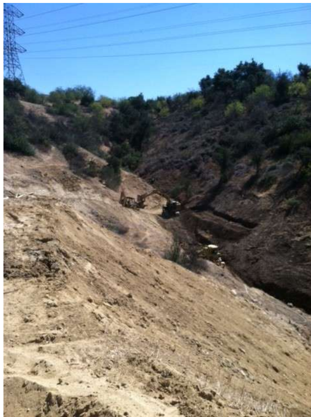
Figure 4: Grading access road to Tower M57-1 in Segment 8 Phase 1, Tonner Canyon.
