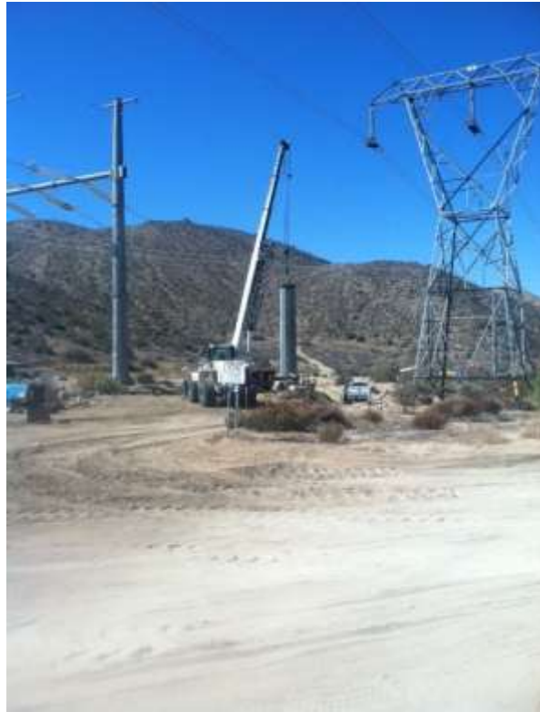
Figure 1: Structure erection occurring at Construct 12 on Segment 6.
