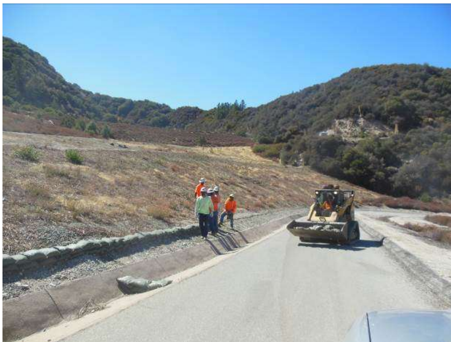
Figure 2: Warren James crew removing sandbag BMPs at Cogswell HAY.
