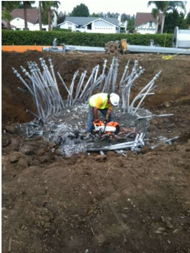
Figure 5: Tower foundation removal in Chino Hills.
