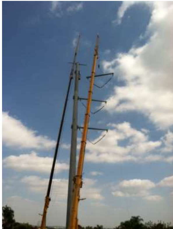
Figure 6: Tower demolition in Chino Hills.
