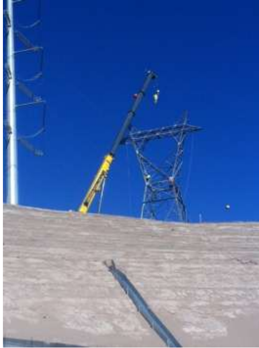
Figure 1: Construct 5 tower wreck-out on Segment 6.
