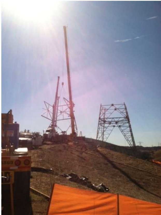
Figure 6: Tower demolition in Chino Hills.
