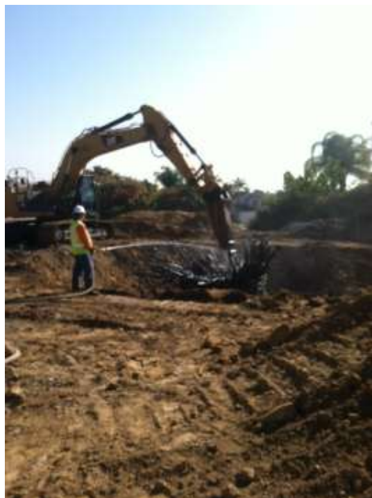
Figure 4: Foundation removal in Segment 8 Chino Hills.
