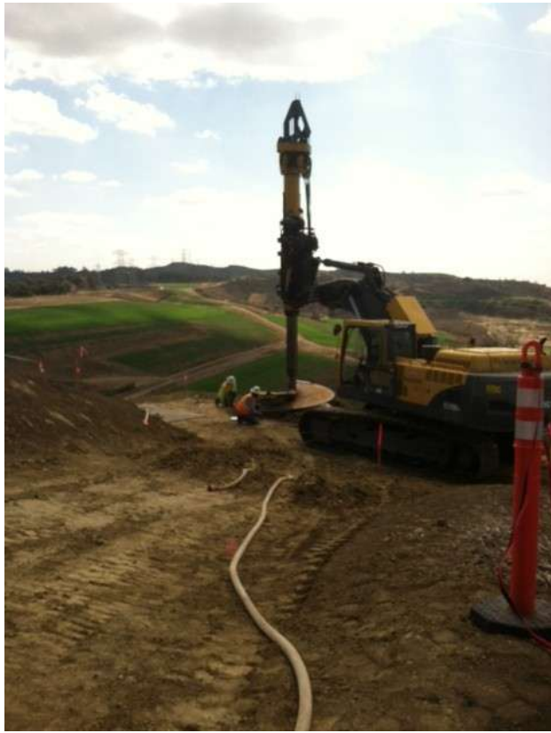
Figure 7: Foundation drilling in Segment 8, Phase 4.
