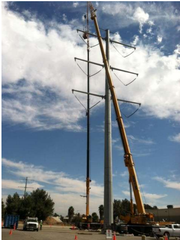
Figure 5: Tower removal in Chino Hills.
