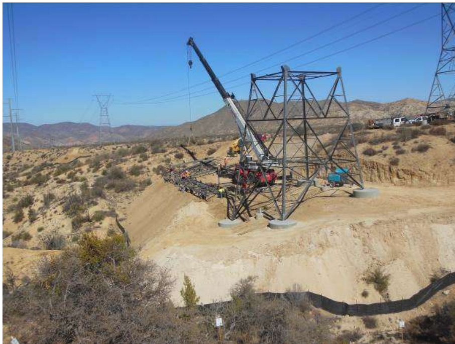
Figure 2: PAR crew assembling tower at Construct 17.
