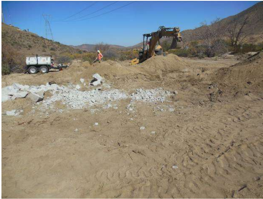
Figure 5: Removal of tower foundations at Construct 11, Segment 6.
