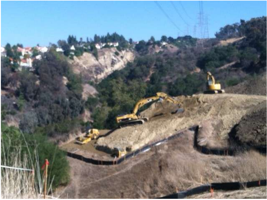
Figure 9: Road construction at Segment 8, Tower M49-T1.
