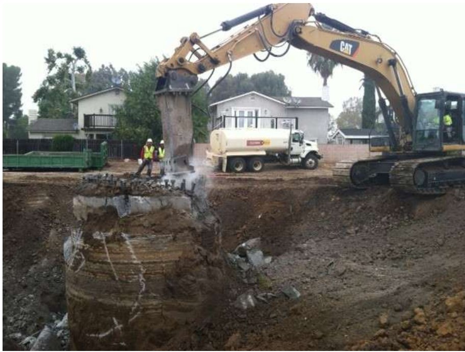
Figure 7: Removal of tower foundations in Chino Hills, Segment 8.
