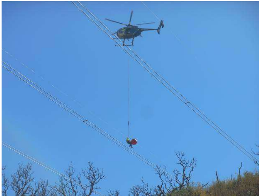
Figure 4: Installation of FAA marker balls between Constructs 23 and 24, Segment 6.
