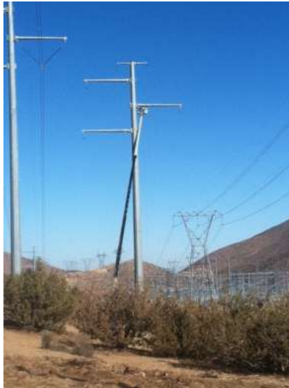
Figure 1: Structure erection at Construct 4 on Segment 6.
