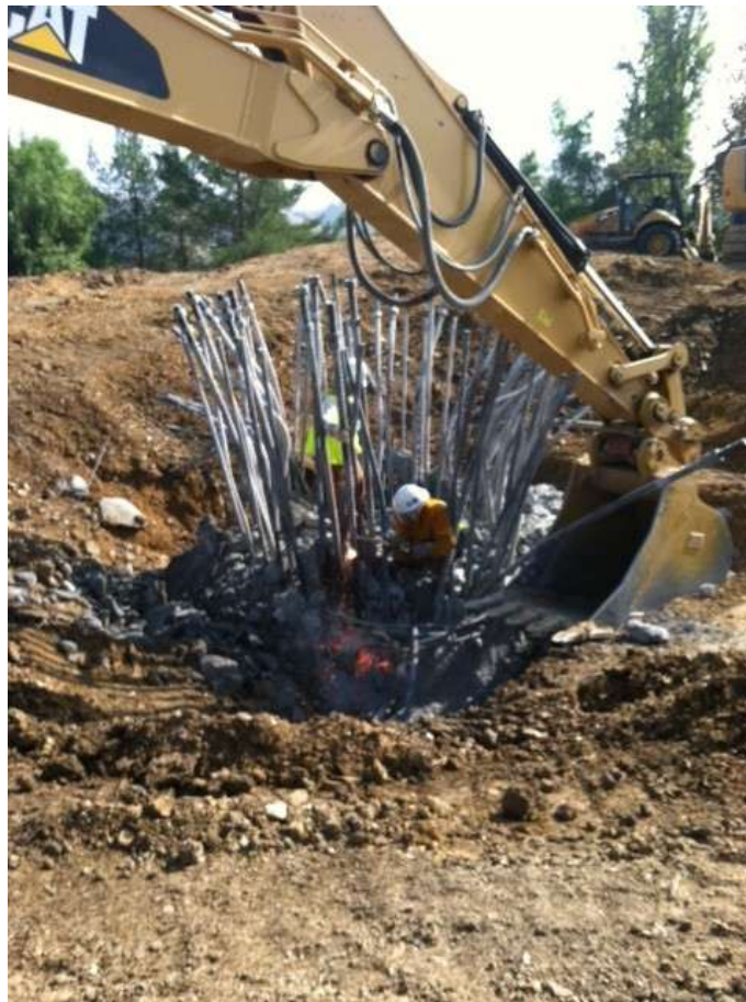
Figure 6: Removal of tower foundations in Chino Hills, Segment 8.
