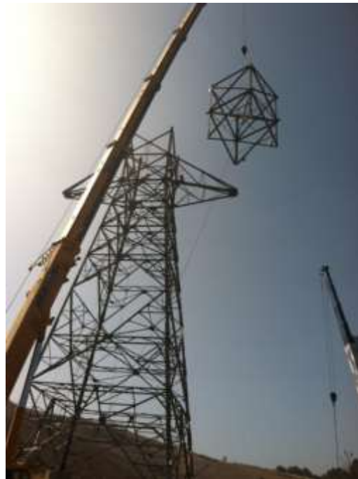
Figure 8: Removal of lattice tower M60-T2 in Chino Hills, Segment 8.
