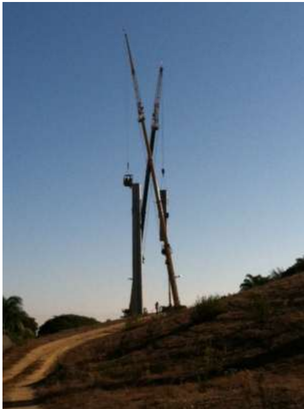
Figure 8: TSP removal in Chino Hills, Segment 8.
