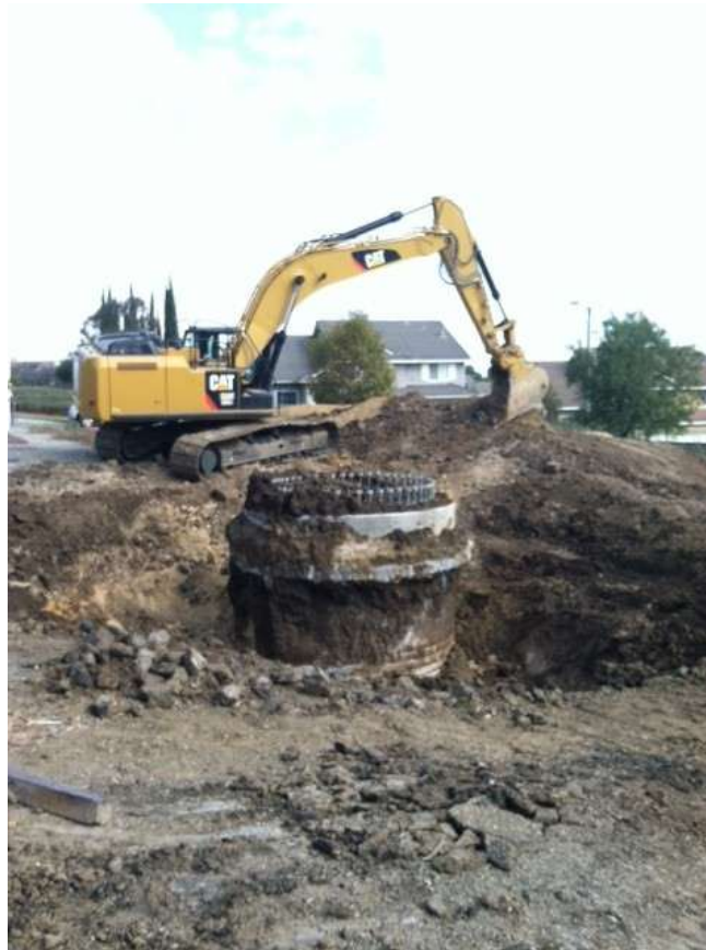
Figure 6: Foundation removal in Chino Hills, Segment 8.
