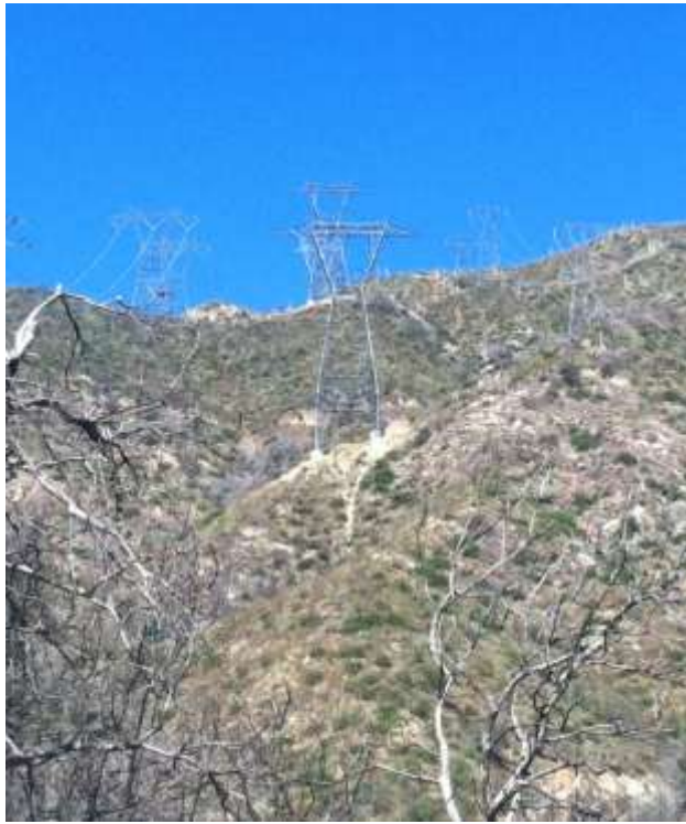
Figure 3: Construct 76 on Segment 6 awaiting the re-installation of perimeter controls.
