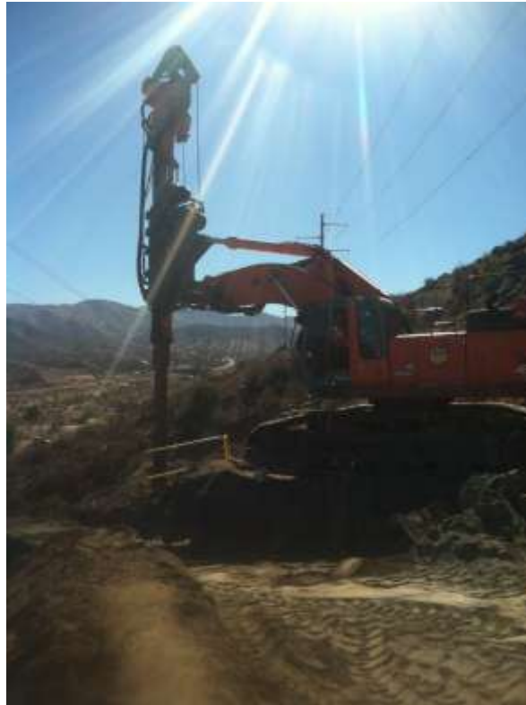
Figure 1: Foundation activities occurring at Construct 8 on Segment 6.
