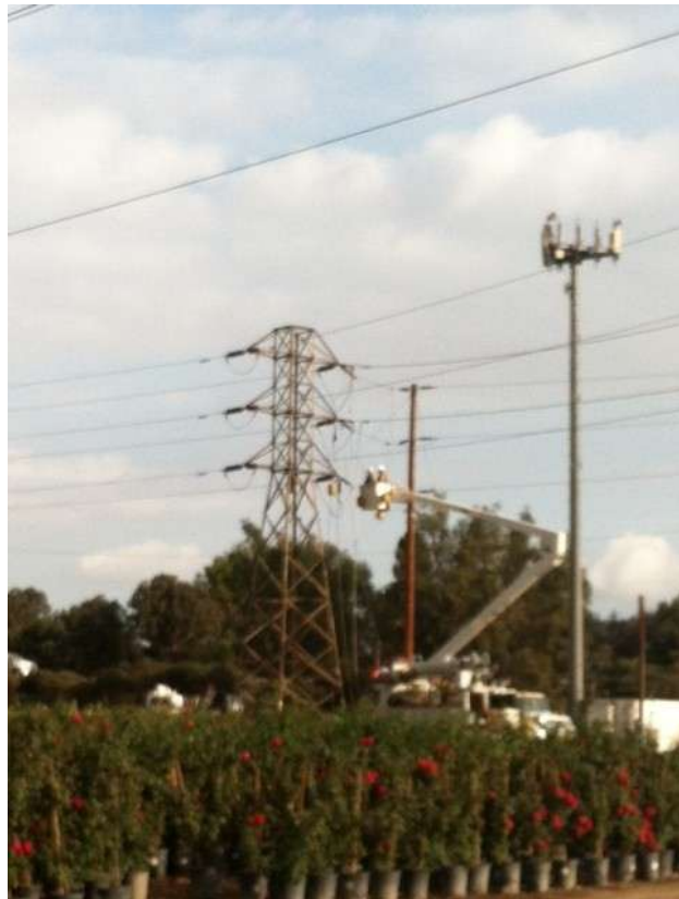
Figure 4: SCE crews stringing towers along the 605 Freeway, Segment 7 66-kV.
