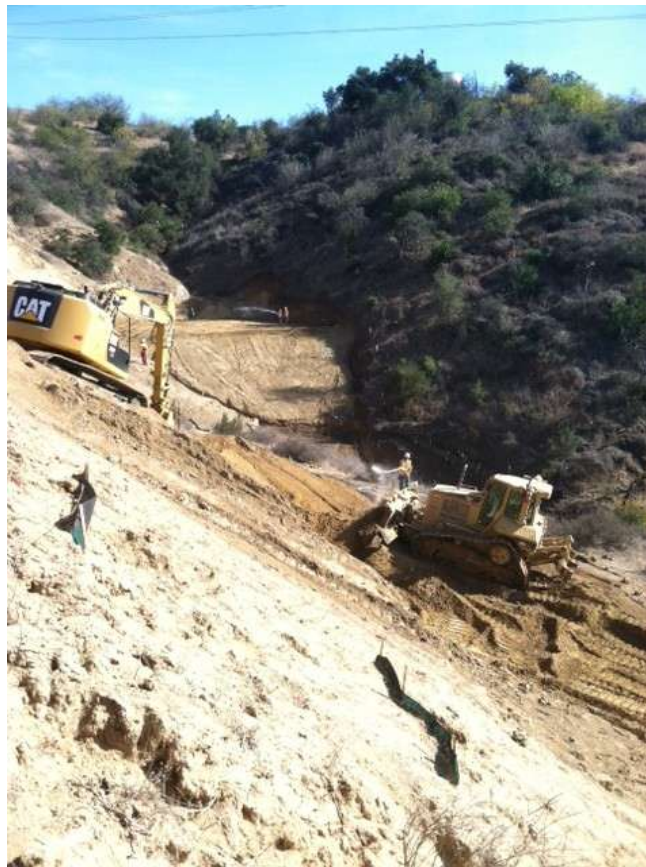
Figure 6: Grading access road to Segment 8, Tower M57-T1, in Tonner Canyon.
