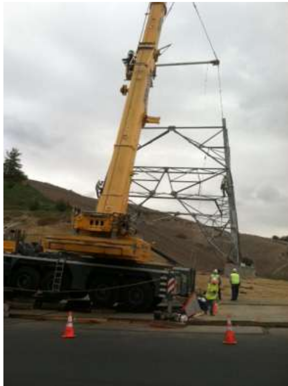
Figure 7: Removal of lattice tower in Chino Hills, Segment 8.
