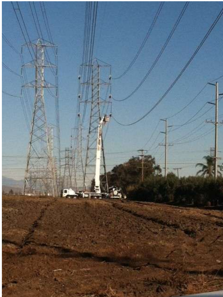
Figure 8: Skyline relocation in Segment 8 Phase 3, in Chino.
