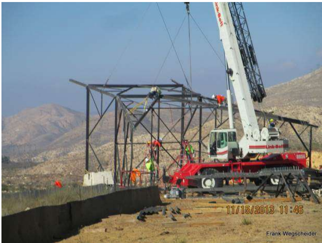
Figure 5: Tower section assembly at the Aliso HAY (photo courtesy of FRED).
