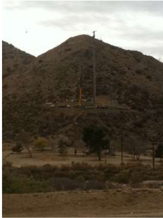
Figure 1: Erection of a tubular steel pole occurring at Construct 9 on Segment 6.
