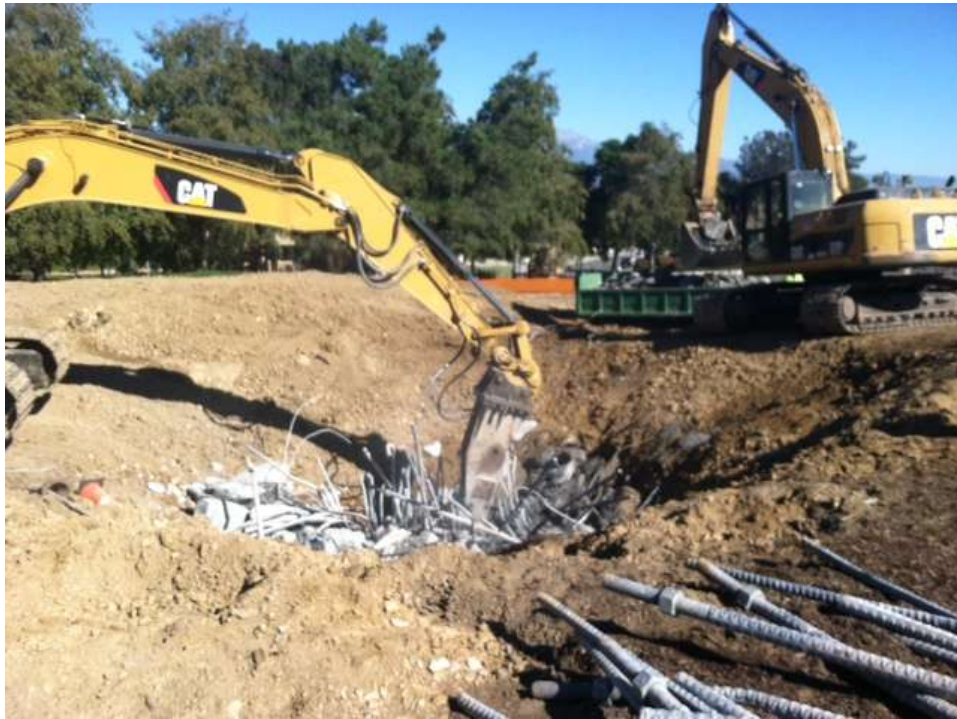
Figure 7: Foundation removal in Chino Hills, Segment 8.
