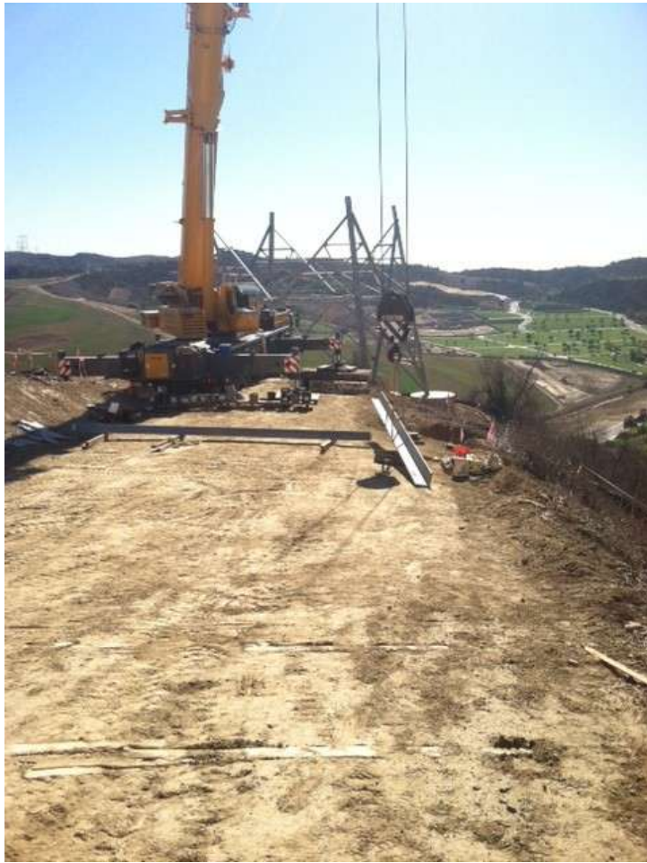
Figure 11: Assembly of Tower 44/3, Segment 8, Phase 4.
