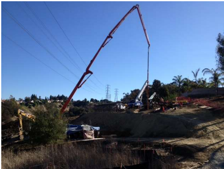
Figure 10: Foundation pouring at Tower 49/1, Segment 8, Phase 4.
