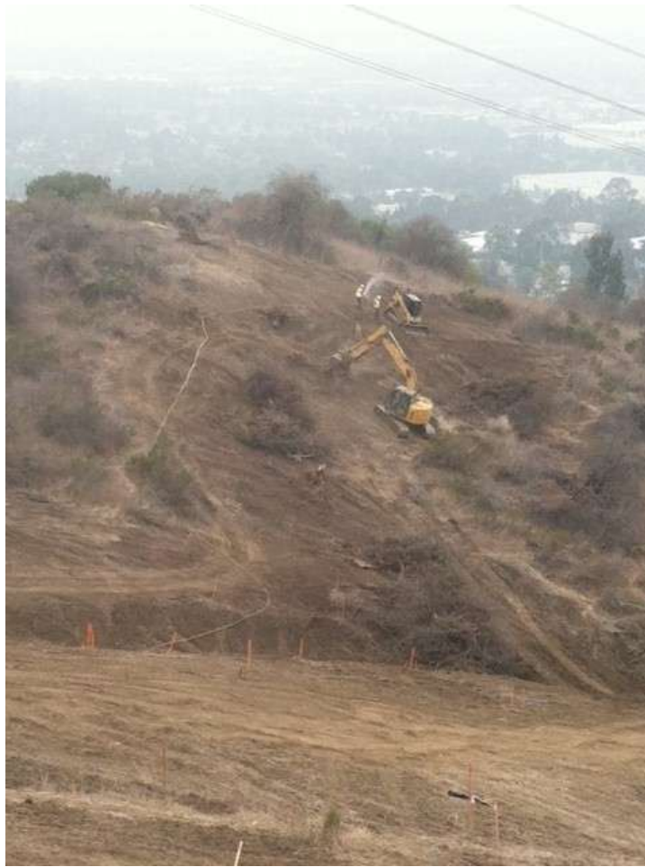
Figure 9: Construction of access road to Tower 43/3, Segment 8, Phase 4.
