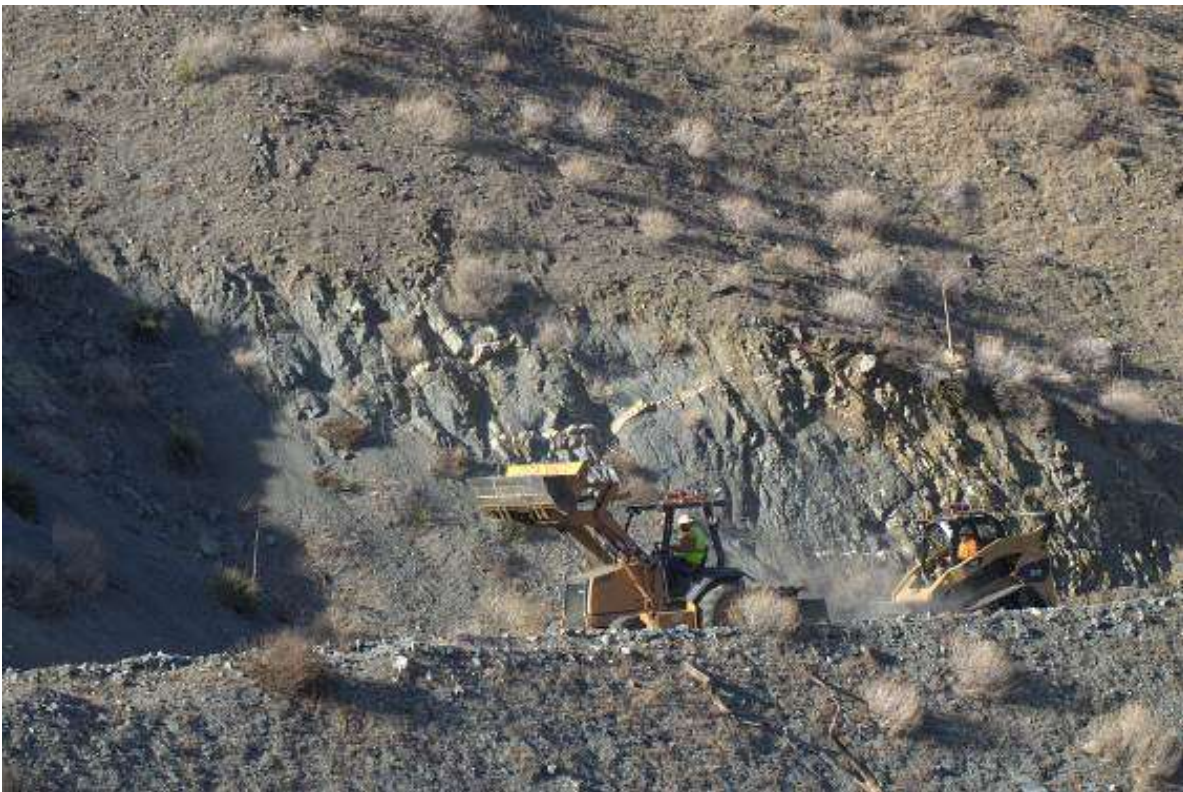
Figure 4: Access road grading between Construct 5 and 11, Segment 11 (photo courtesy of FRED).
