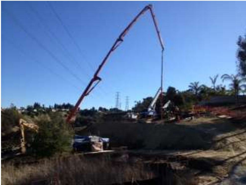
Figure 5: Concrete foundation pouring at Tower M49-T1, Segment 8.
