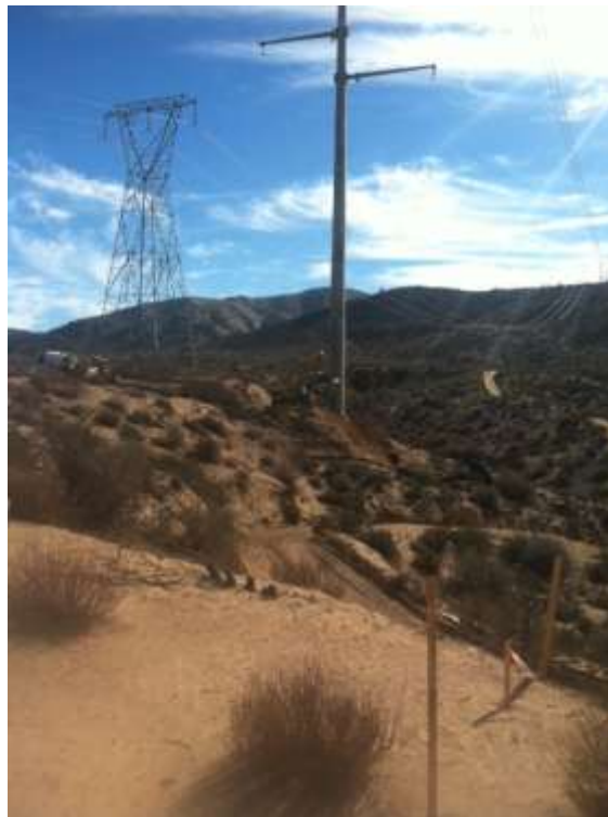
Figure 2: Construct 16 grading activities, Segment 6.
