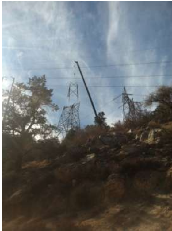
Figure 1: Construct 19 erection activities, Segment 6.
