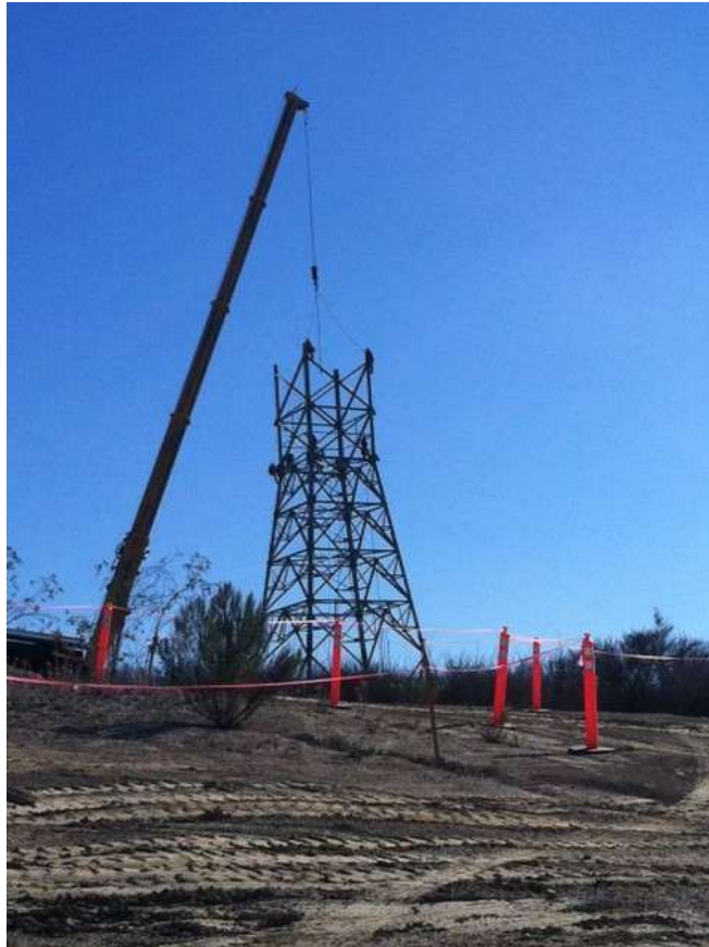
Figure 6: Tower M44-T3 assembly, Segment 8.
