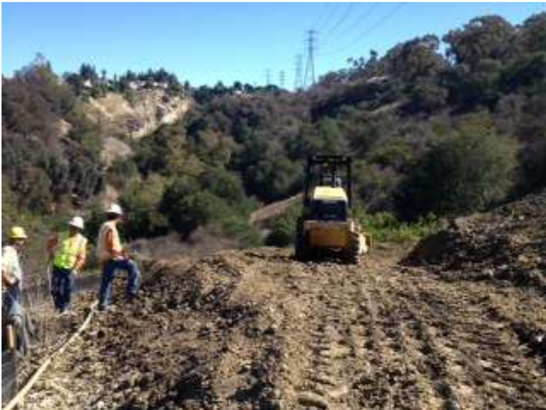
Figure 4: Grading of tower site, Segment 8, Tower M49-T1.
