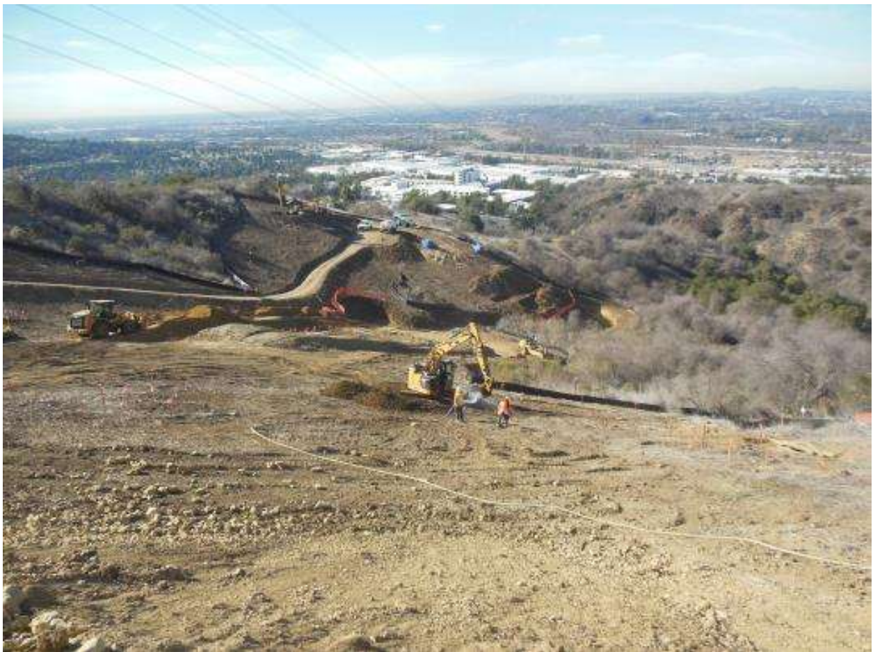
Figure 8: Grading work area at Segment 8, Phase 4, Tower M43-T3.
