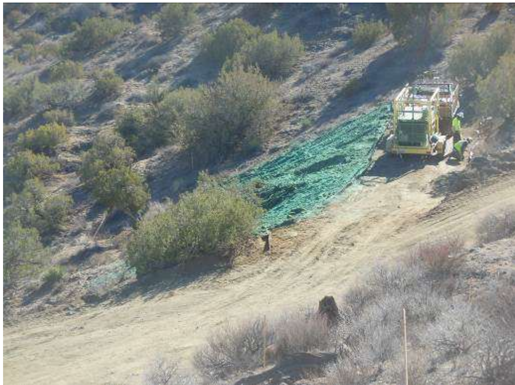
Figure 2: Hydromulching at Construct 5 on Segment 11C.
