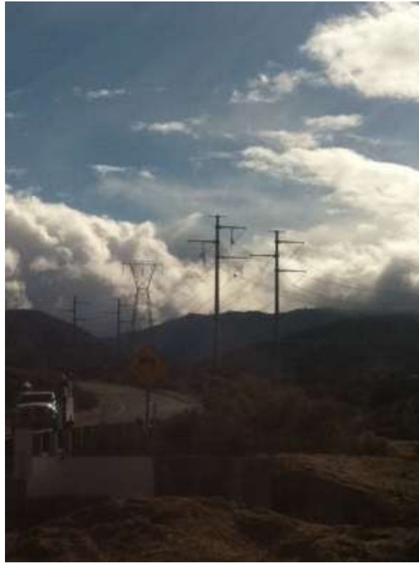
Figure 1: Construct 14 wire stringing activities, Segment 6.
