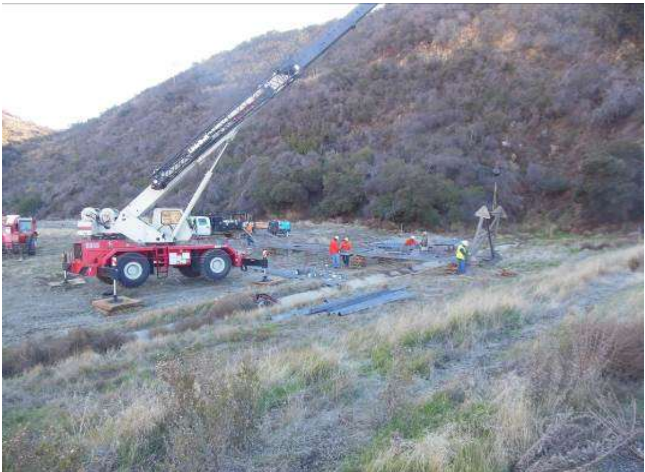
Figure 4: Assembly crews onsite at the Maple Canyon HAY.
