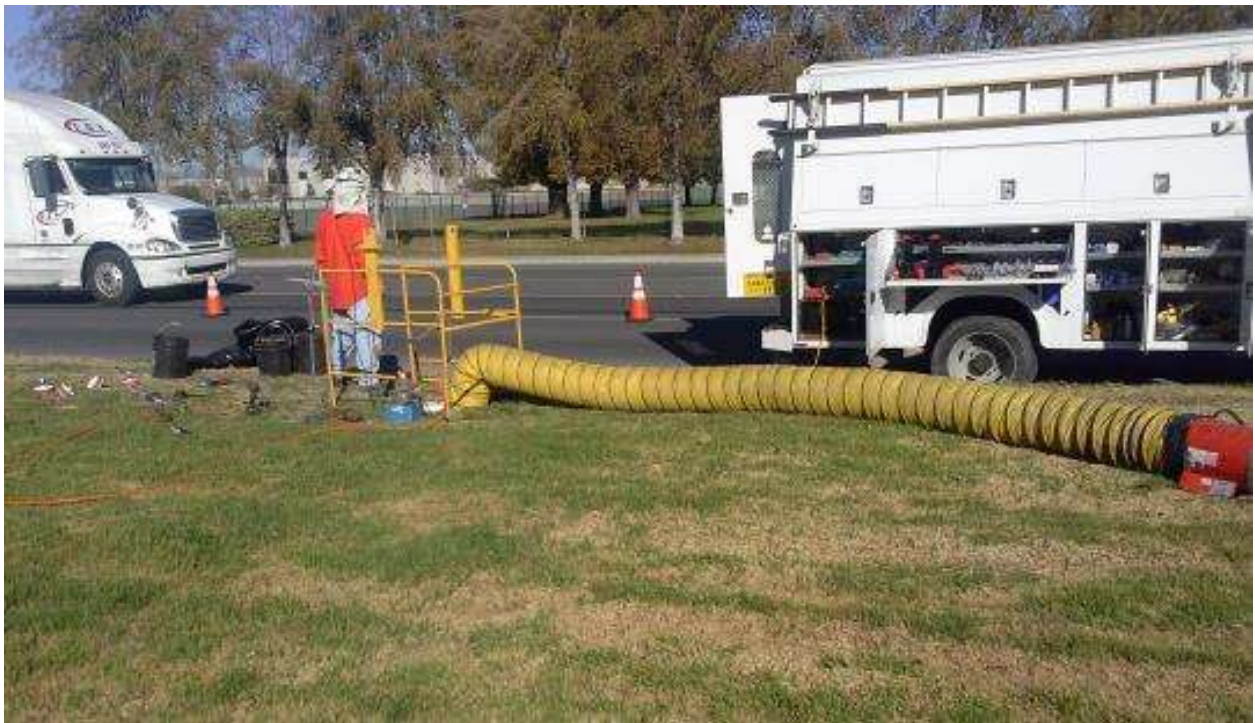
Figure 7: 66 kV underground cable installation at Ayala Park, City of Chino.
