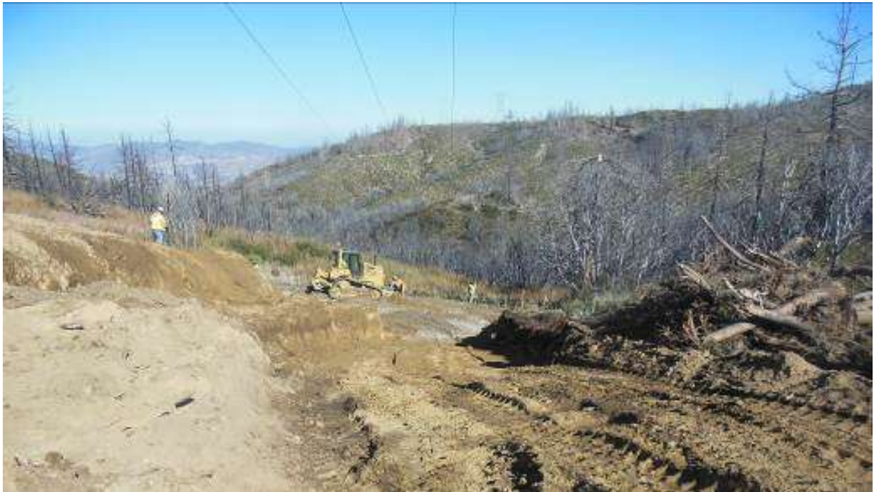
Figure 3: Grading keyway at Construct 31 on Segment 11C.
