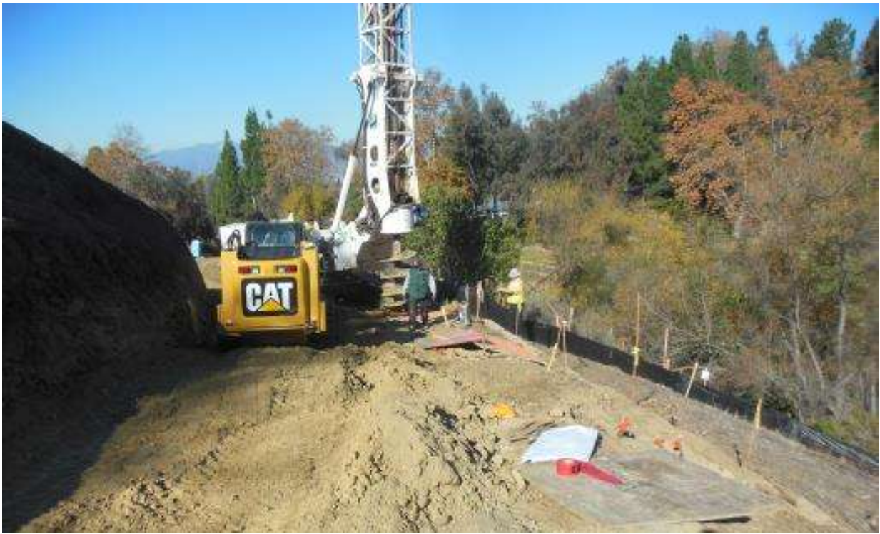
Figure 9: Soldier pile wall foundation work at Tower M49-T1, Segment 8, Phase 4.
