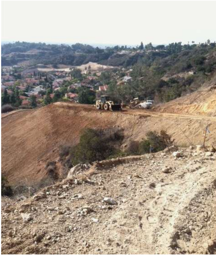
Figure 5: Grading access road to Tower M27-T3 in Duarte.
