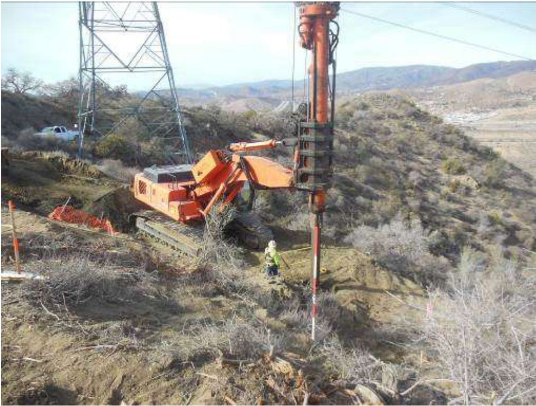
Figure 3: Foundation drilling at Construct 4 on Segment 11C.
