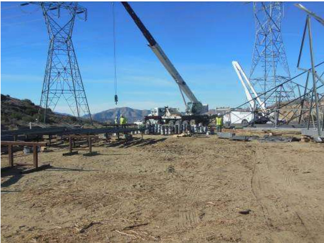
Figure 4: Assembly crews onsite at Construct 1 on Segment 11C.
