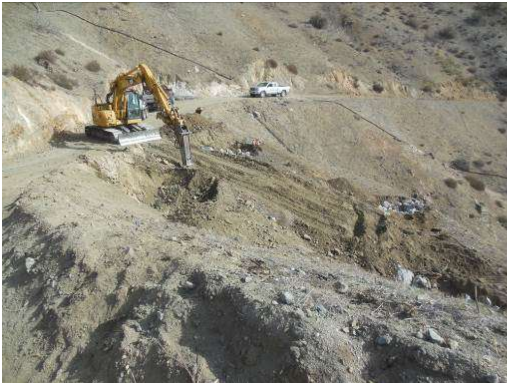
Figure 2: Removal of existing concrete foundations at Construct 8 on Segment 11C.
