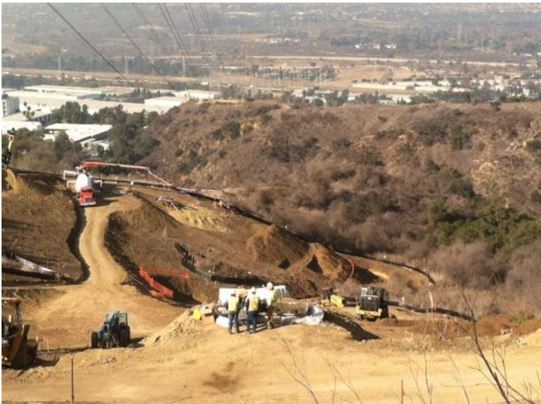
Figure 6: Pouring foundations at Tower M43-T3.
