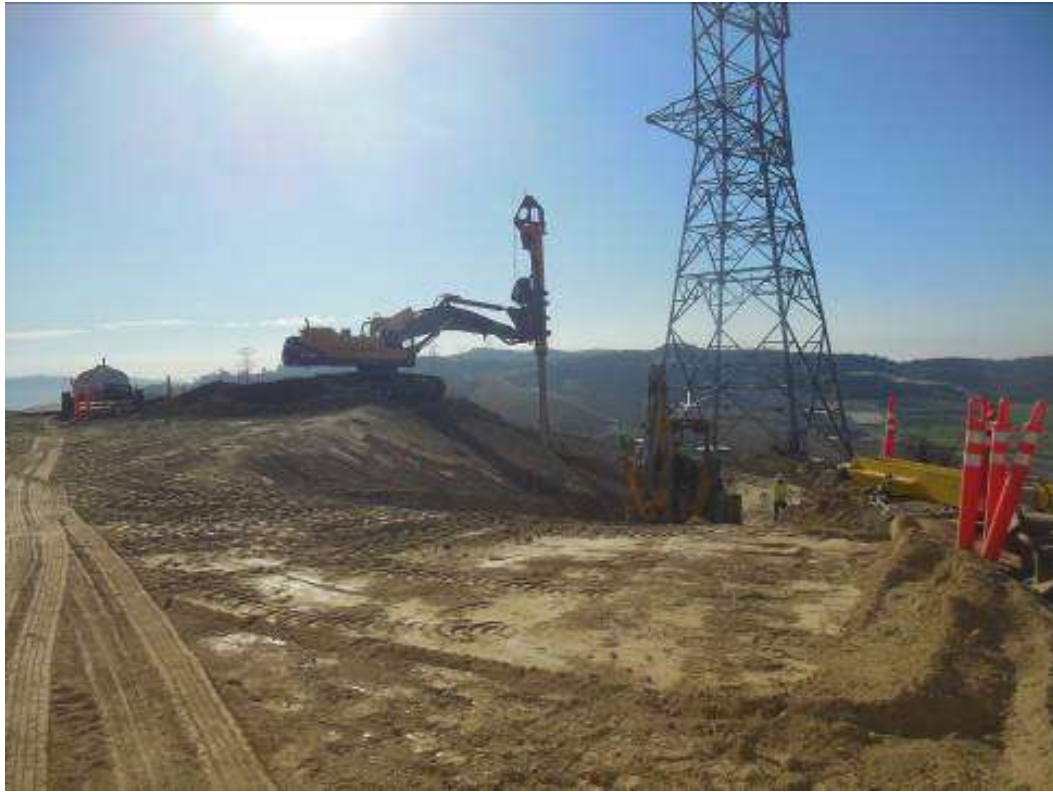
Figure 6: Foundation drilling by kV Structures at Tower M44-T3, Segment 8, Phase 4.
