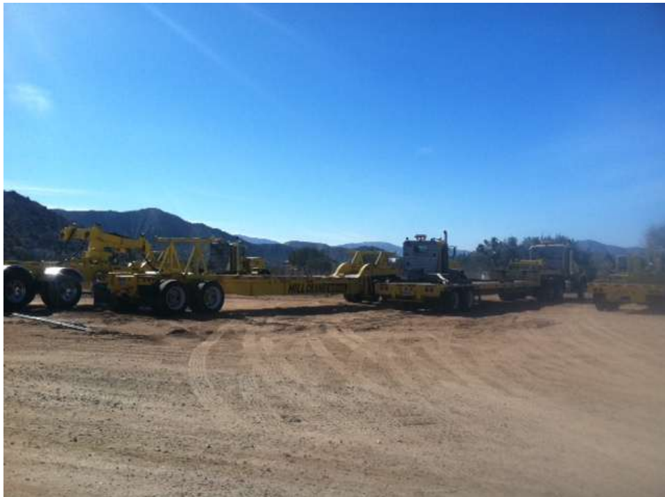
Figure 2: Staged trucks, associated with work at Construct 1 on Segment 6, within an area not approved for disturbance.
