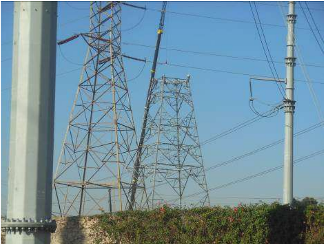
Figure 8: Assembly activities at Tower M9-T3A, Segment 8, Phase 4.
