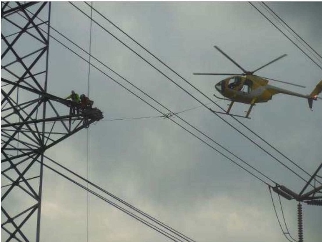
Figure 8: Helicopter pulling wire through traveler at Tower M42-T3, Segment 8, Phase 4.
