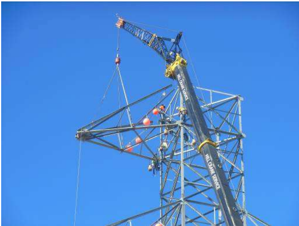
Figure 6: Installing an arm at Tower M37-T4, Segment 7.
