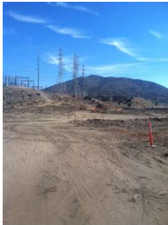
Figure 2: Grading activities occurring at Construct M0-T1, Segment 11C.
