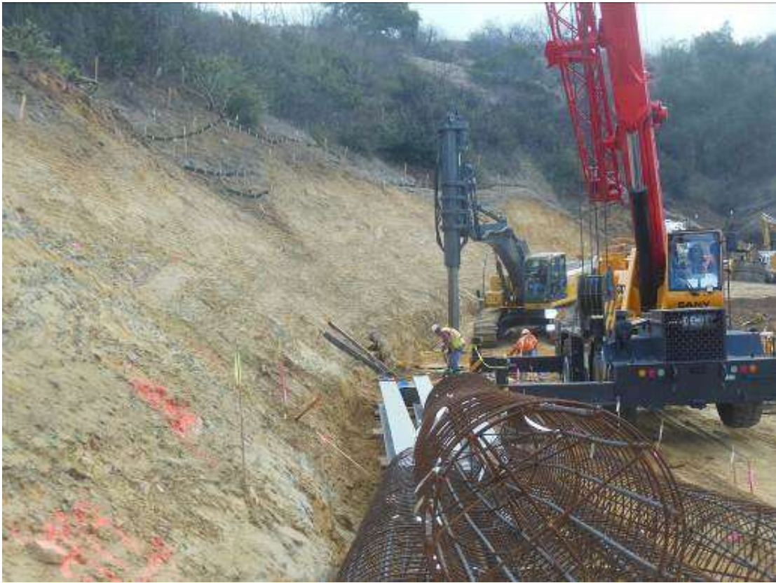
Figure 7: Drilling hole for retaining wall foundation at Tower M57-T1, Segment 8, Phase 1.
