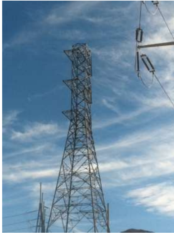
Figure 1: Steel inspection for wire activities occurring at Construct 2, Segment 6A.
