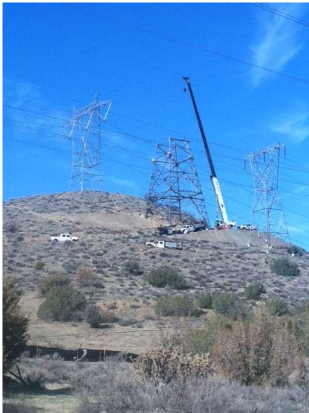
Figure 3: Erection activities occurring at Construct 4, Segment 11C.
