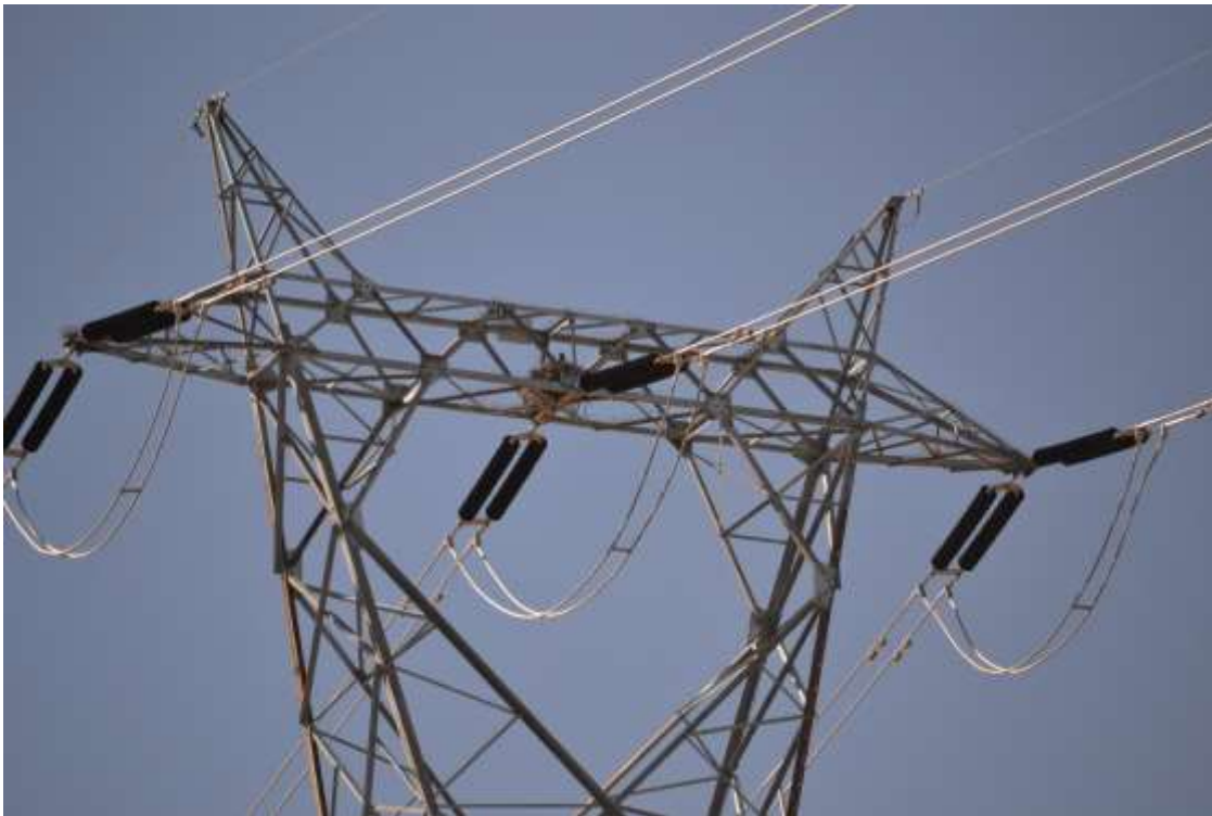
Figure 4: SCE requested a reduced construction buffer for a red-tailed hawk nest on Segment 11C.
