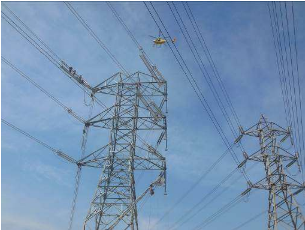
Figure 8: Final stages of wire installation at Tower M41-T2, Segment 8, Phase 4.
