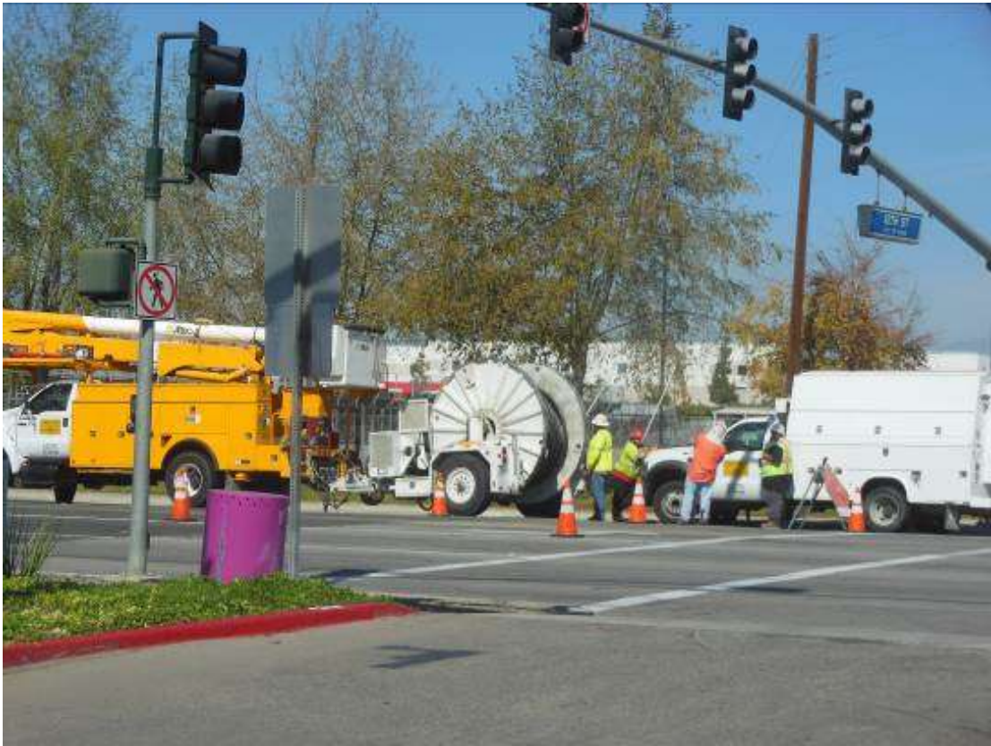
Figure 5: Ongoing 66 kV work in the City of Chino, Segment 8 66 kV.
