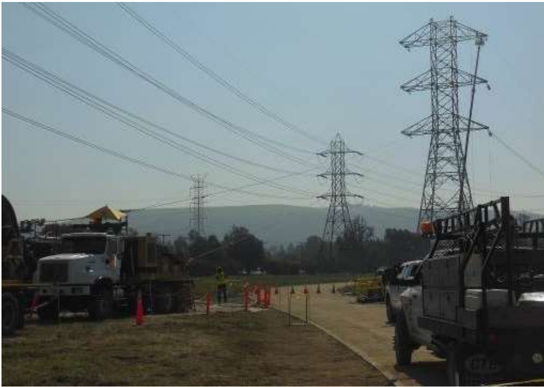
Figure 5: Wire pulling operations occurring between Towers M36-T2 and M37-T3, Segment 7.
