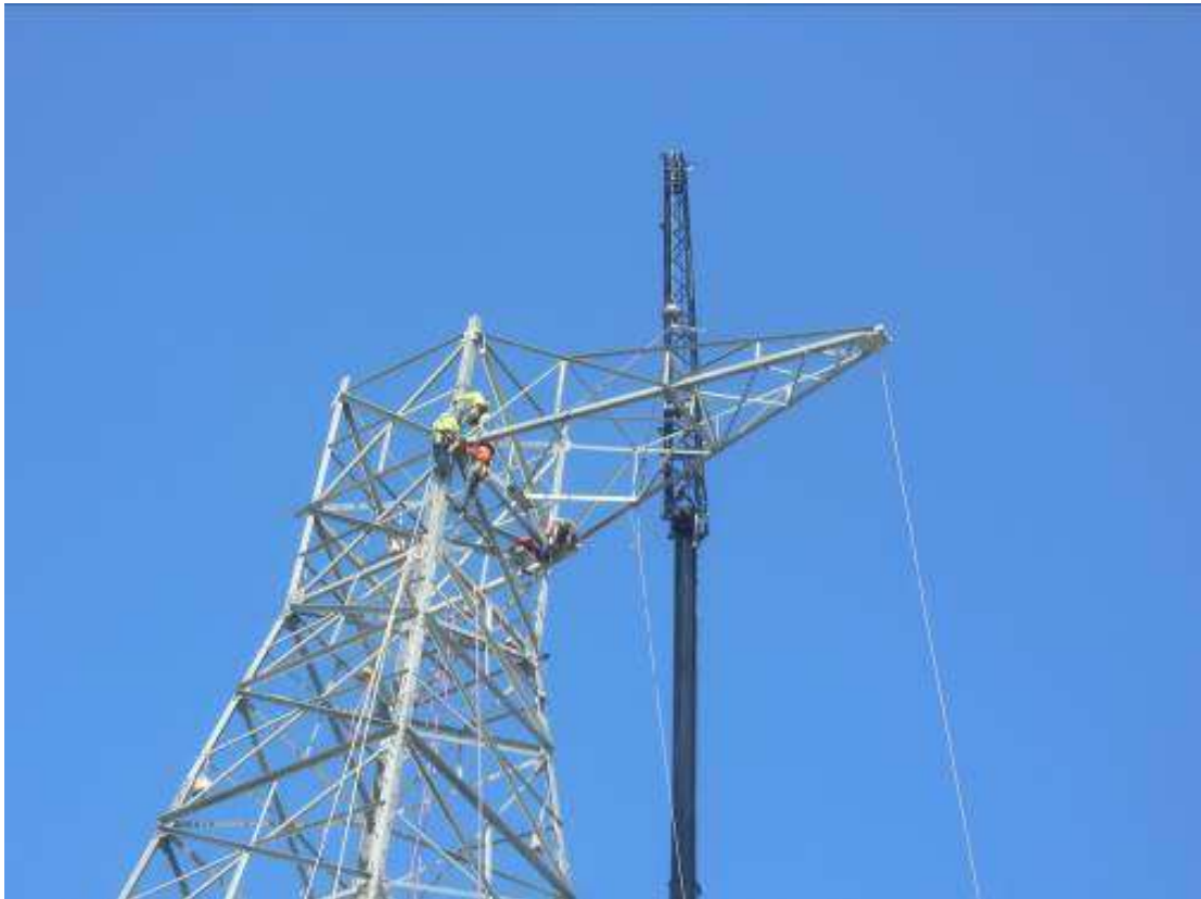
Figure 4: Assembly crews installing arm at Tower M35-T3, Segment 7.
