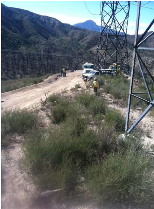
Figure 2: BMP removal occurring at Construct 63, Segment 6B.
