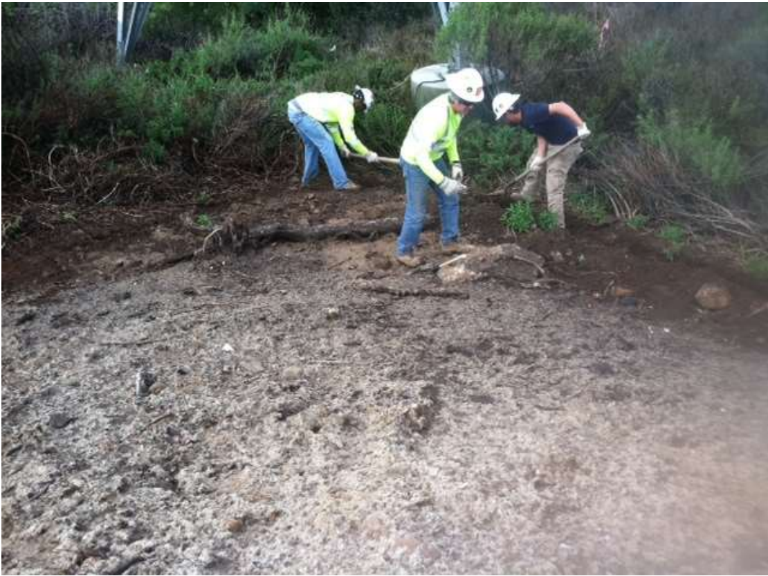
Figure 3: Silt fence installation occurring at Chaney Trails pull site, Segment 11B.
