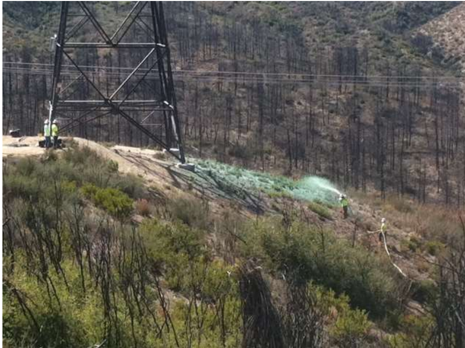
Figure 1: Crews spraying hydromulch at Construct 63, Segment 6B.
