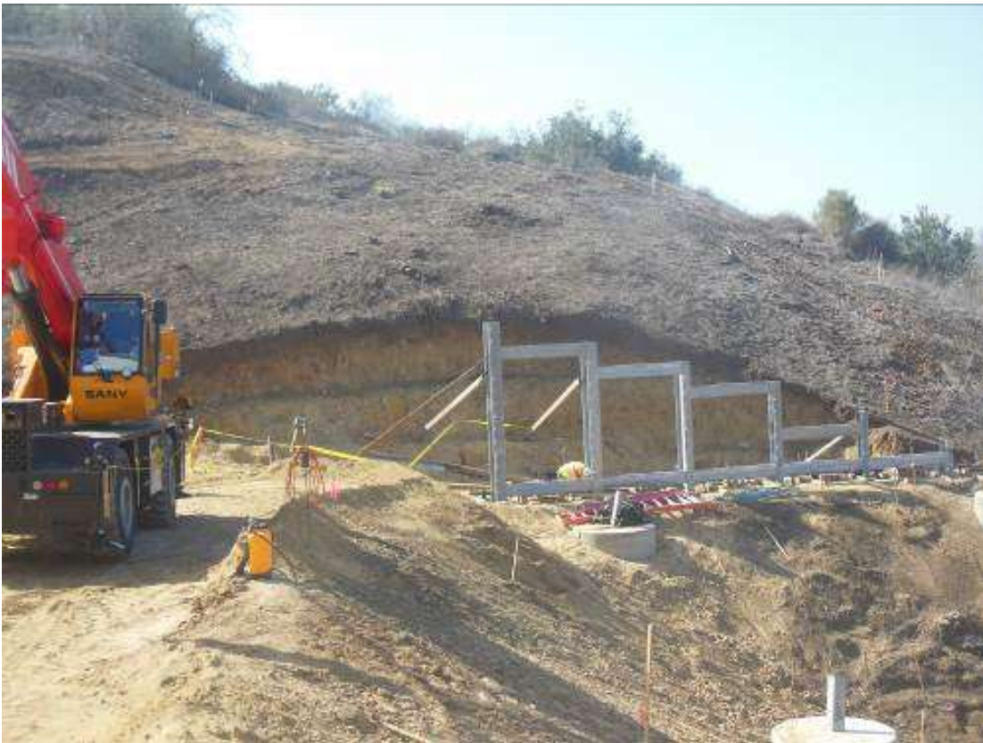
Figure 6: Installation of the southern retaining wall at Tower M57-T1, Segment 8, Phase 1.
