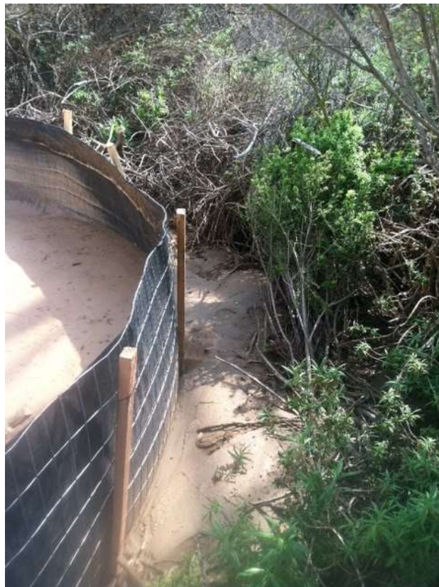
Figure 2: Sediment flow beyond the site boundary at Chaney Trails Pull Site, Segment 11B.
