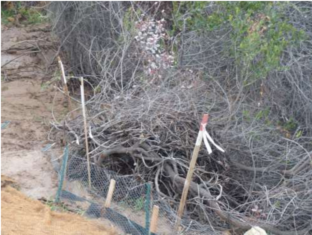
Figure 10: Post storm inspections identified multiple locations where sediment overtook BMPs and traveled off site into a woodrat midden, Tower M27-T3 (photo courtesy of FRED).
