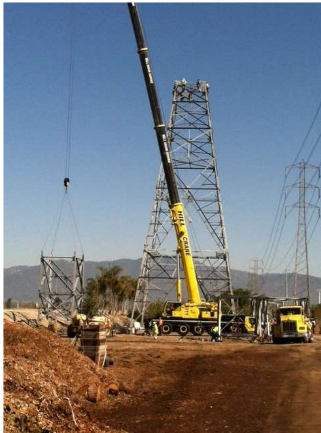
Figure 3: Tower assembly on Segment 7.
