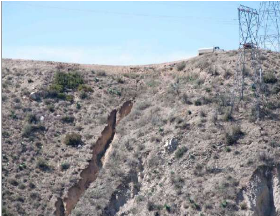
Figure 2: Offsite erosion after early March storm at Tower 54, Segment 11C.
