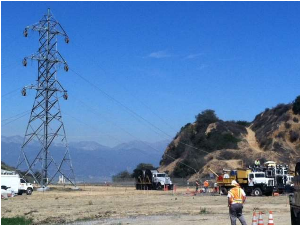
Figure 5: Wire stringing activities near Rose Hills, Segment 8, Phase 4.
