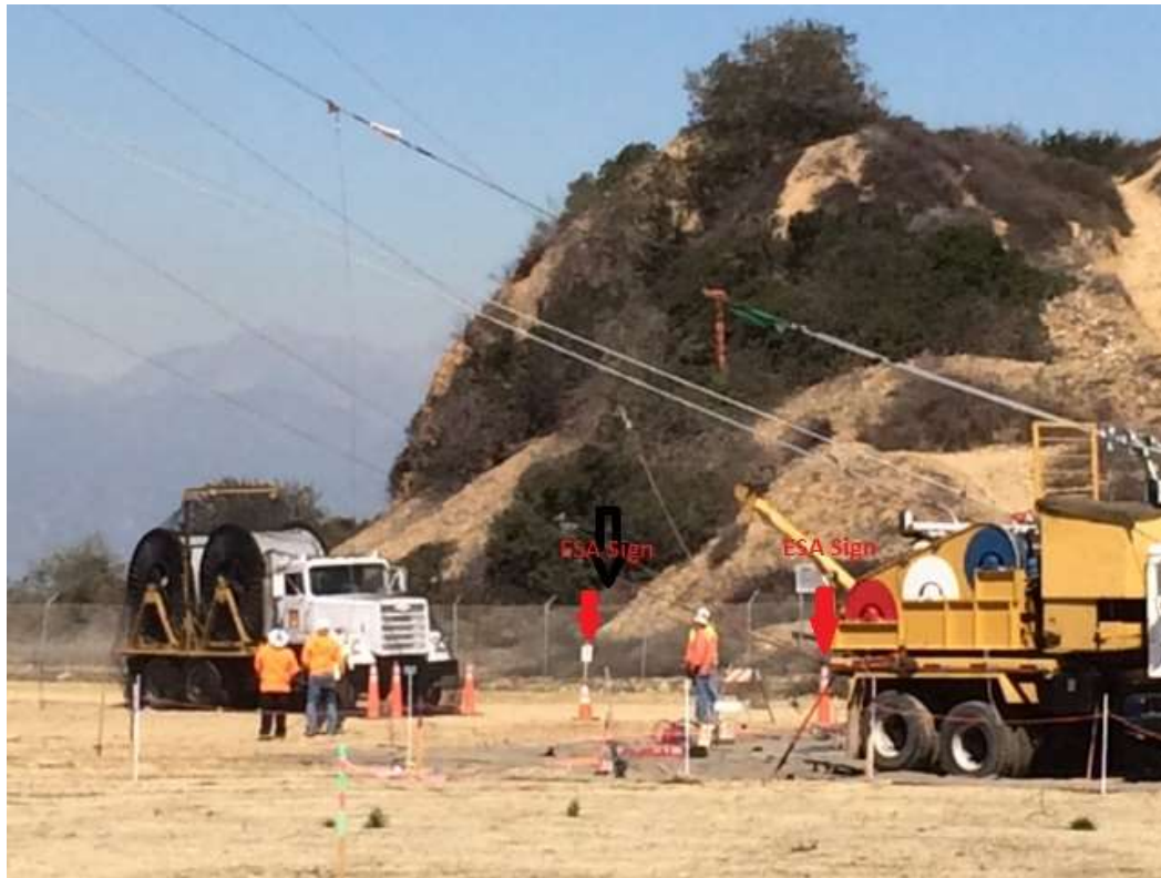
Figure 6: PAR crews staged equipment within a clearly marked ESA, Segment 8, Phase 4.
