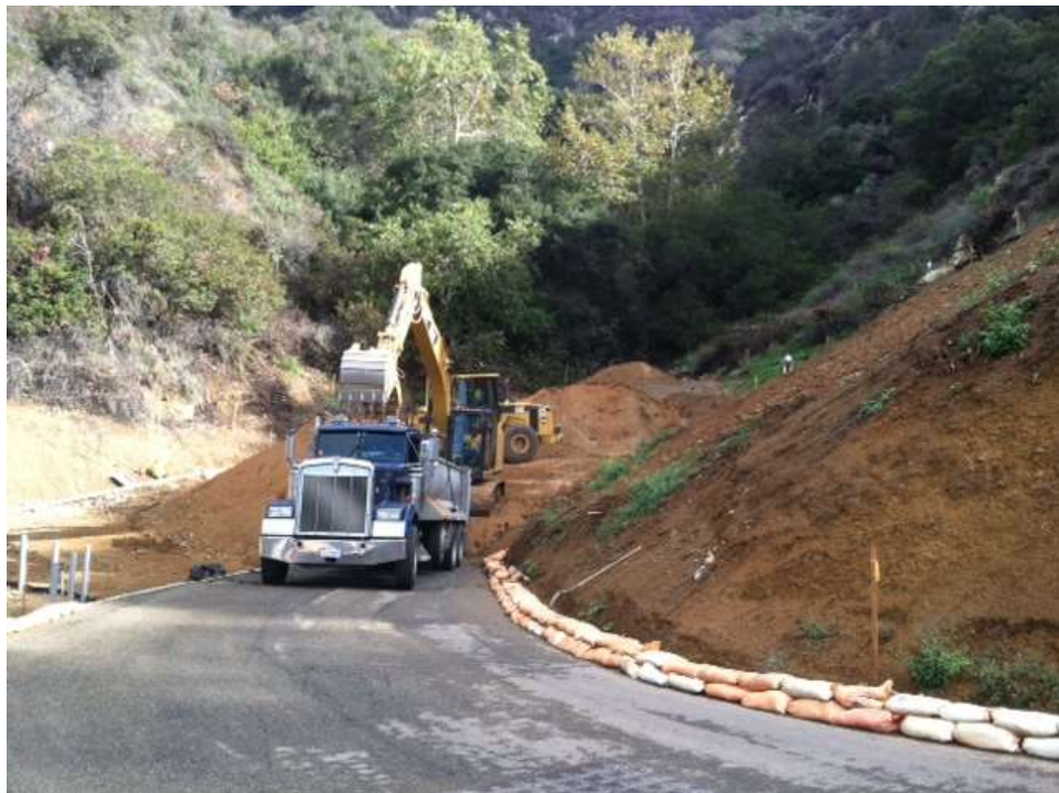
Figure 6: Soil export at M27-T3 in the City of Duarte, Segment 7.
