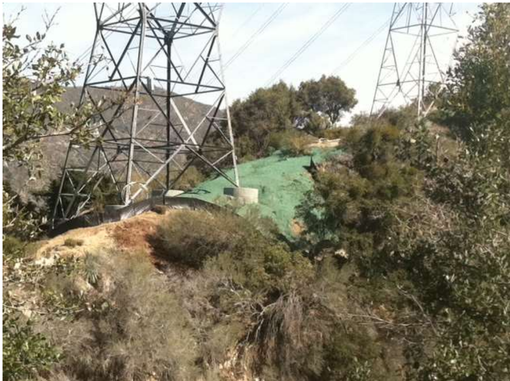
Figure 2: Recently completed hydromulch application at Construct 81, Segment 6C.
