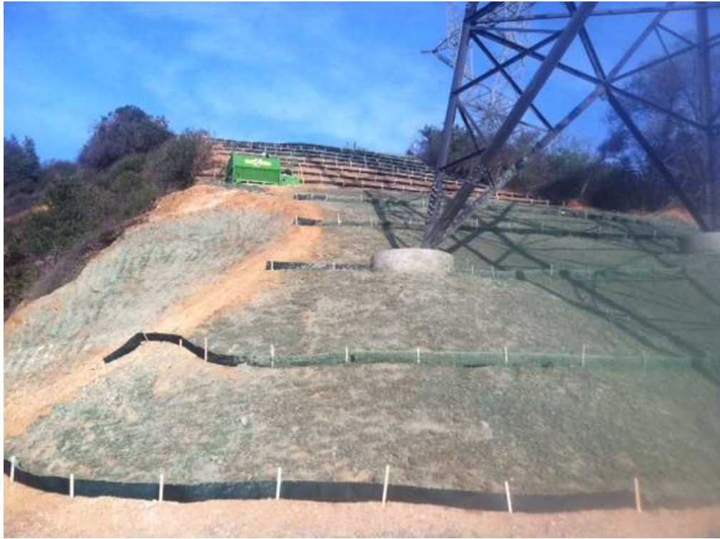
Figure 1: Hydromulch and Prowattle application on the slope of Construct 113, Segment 6C.
